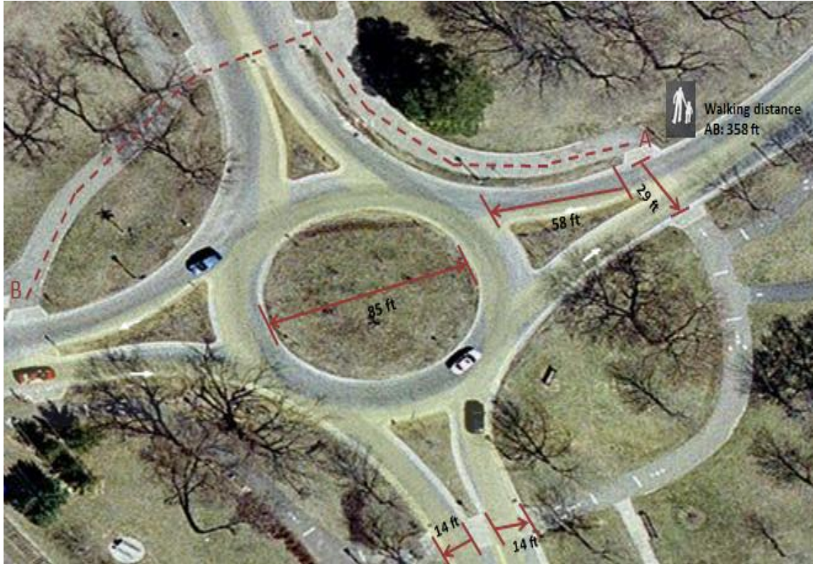
Figure 3-3 Roundabout at Minnehaha Pkwy and Minnehaha Ave
