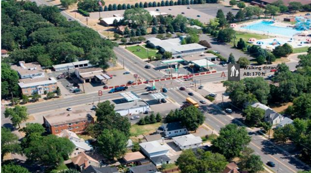
Figure 3-1 66th St and Portland Ave Intersection before the Roundabout Construction
