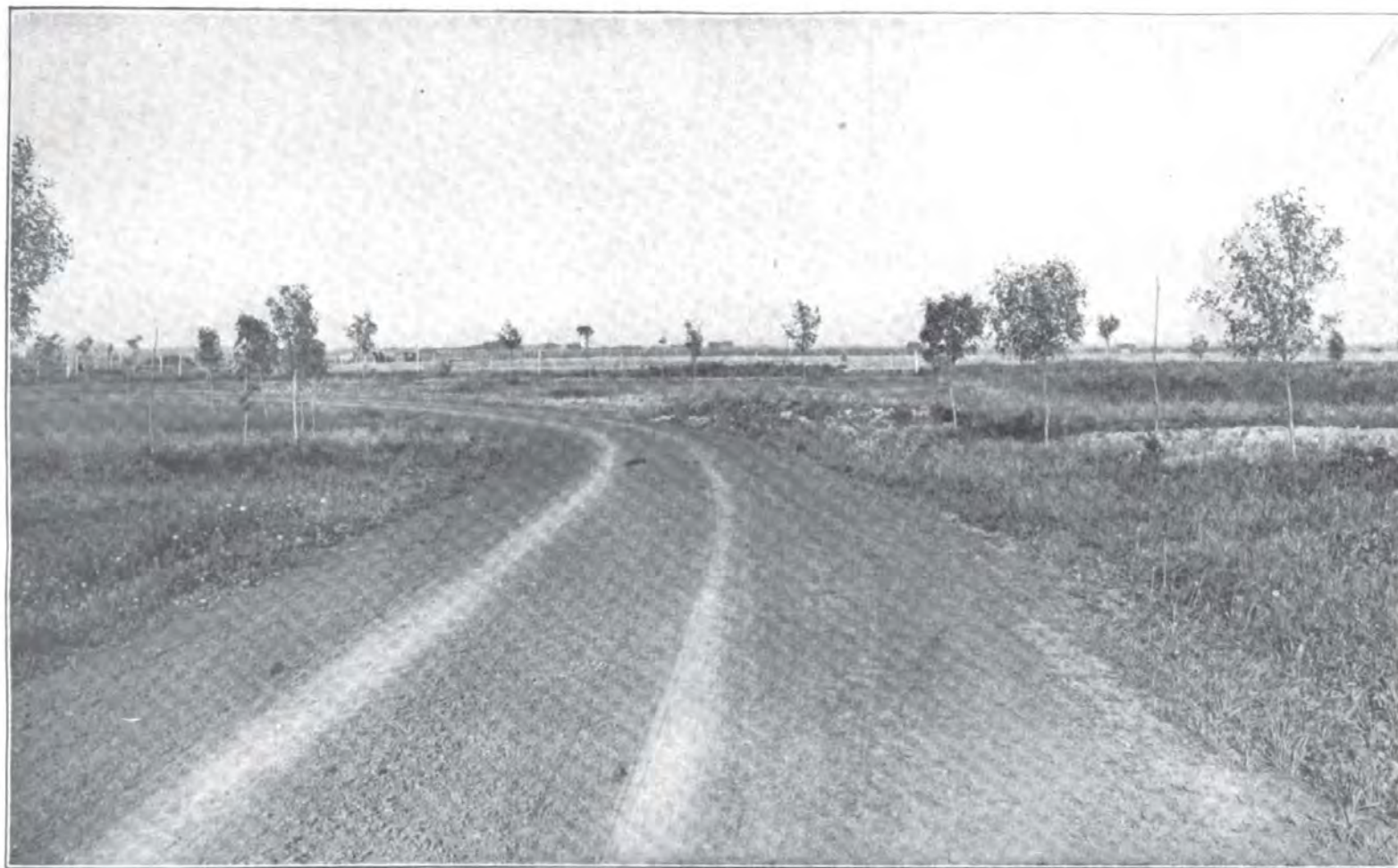
DIRT ROAD AT NORTHWEST EXPERIMENT FARM, CROOKSTON, MINN. KEPT IN REPAIR BY USE OF KING ROAD DRAG AND ONE TEAM.
