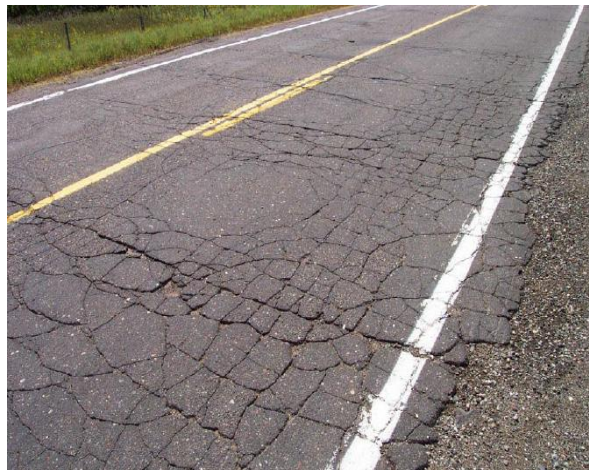
Figure 9. Severely Deteriorated Pavement Surface Condition
