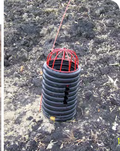
(L) Demonstration site: Slotted riser and gravel inlet. Kandiyohi County, MN. (R) Slotted-raised inlet.
