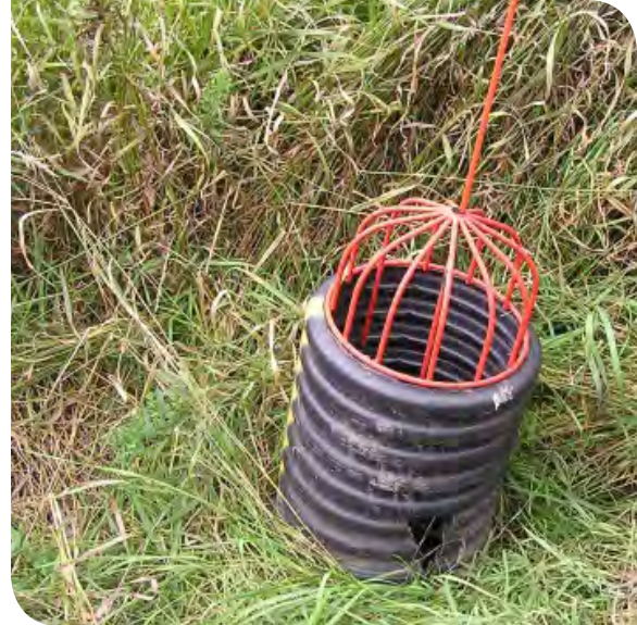
Figure 14. Standpipe side inlet in Kandiyohi County, MN.
