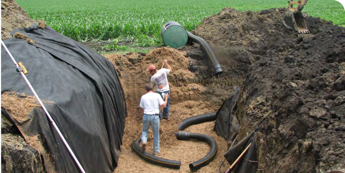
Woodchip bioreactor installation.
