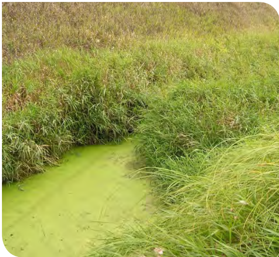
Figure 11. Reduced conveyance due to side inlet failure
