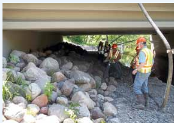
Investigators train MnDOT staff on proper techniques for installing matrix riprap on a bridge abutment.
