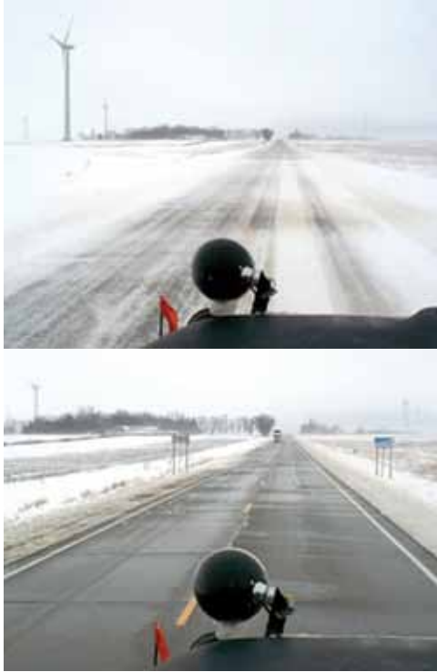
A segment of road with a living snow fence (bottom) offers better driver visibility and road surface conditions than a segment of road without this natural windbreak (top). MnDOT traffic safety data suggest that living snow fences can reduce snow- and ice-related accidents by 40 percent on roadways with super-elevated curves.
