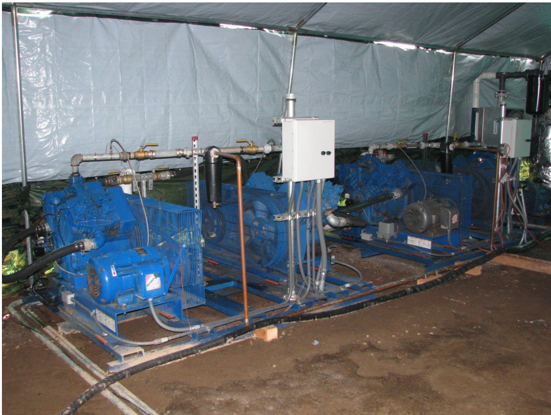
C3 remediation system at the WDE Landfill, Anoka County
