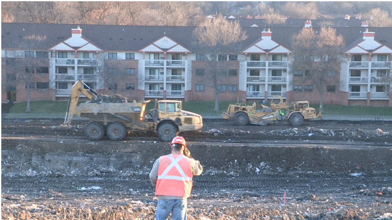
Relocating waste away from adjacent apartments at the Hopkins Landfill, Hennepin County
