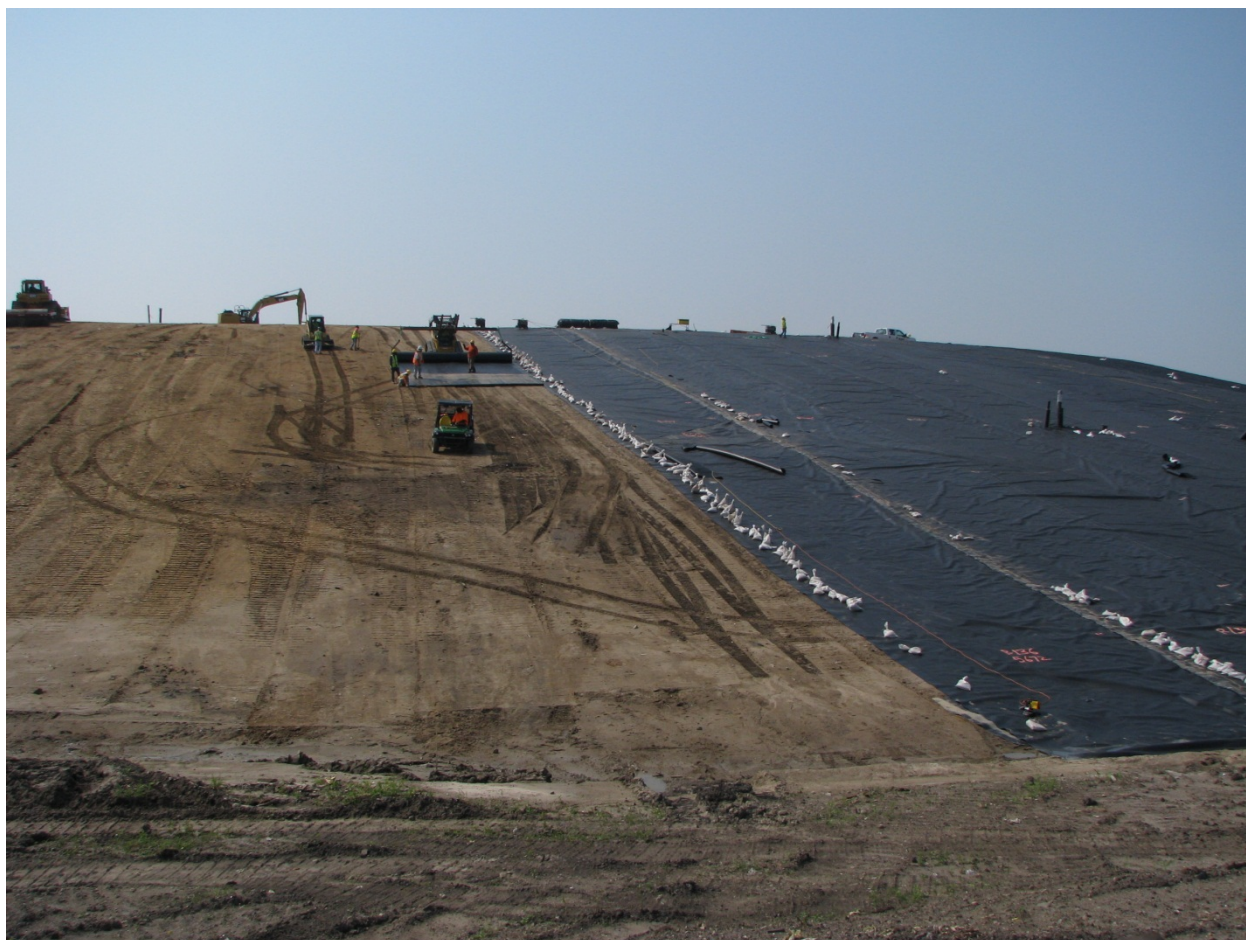
Installing new cover and plastic liner at the Hopkins Landfill, Hennepin County
