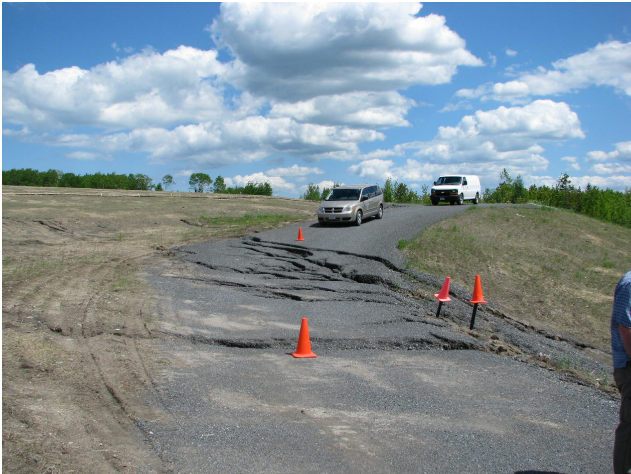
O&M - Road repair needed at the Koochiching County Landfill
