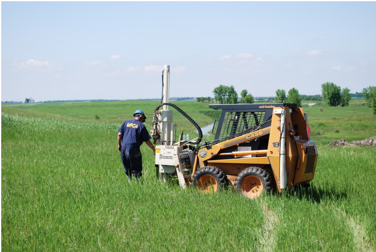
Geoprobng for waste at the Pipestone County Landfill
