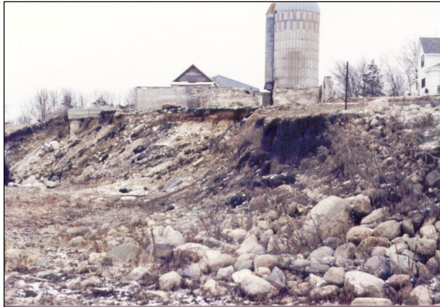
Figure 6. Erosion zone near farm site
