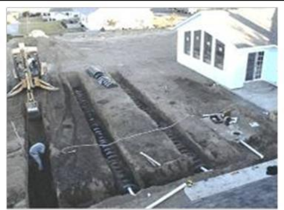
Figure 12. Typical septic system installation
