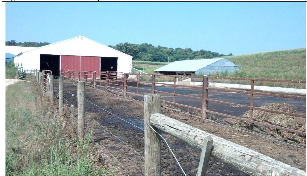
Figure 31. Goodhue Feedlot Improvements.
