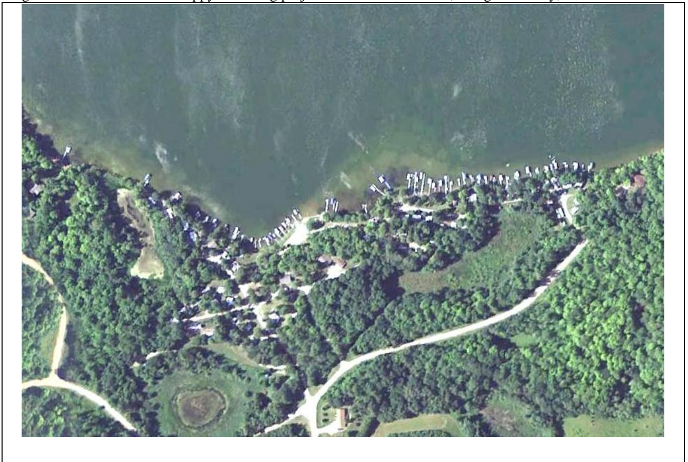
Figure 42. Aerial view of Happy's Landing project site on Lobster Lake, Douglas County, MN.
