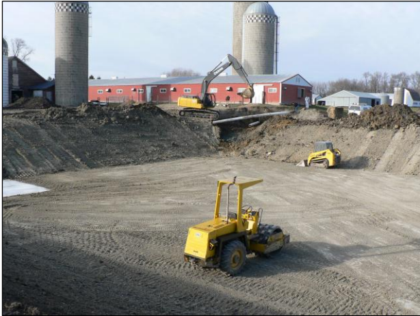
Figure 2. Typical manure storage pit under construction in Stearns County
