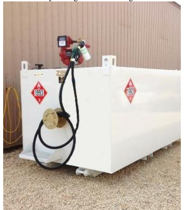
Figure 29. Example of a double wall containment tank funded by the AgBMP Loan Program
