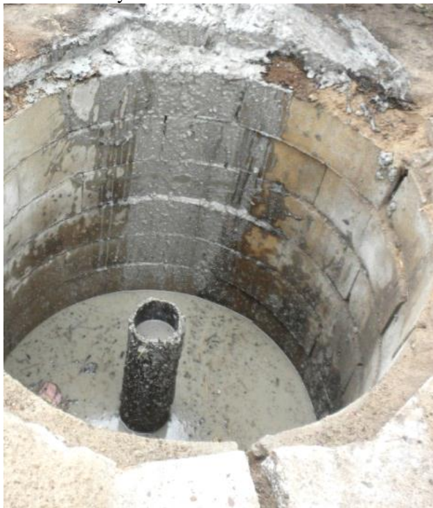
Figure 28. Well sealing project completed in Benton County
