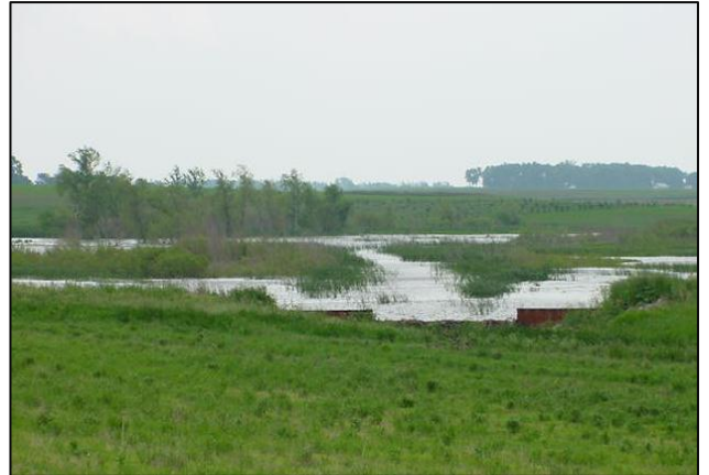
Figure 7. Sediment and water control basin in Lincoln County
