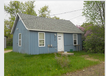
Exterior of Home to be Demolished
