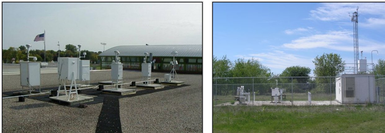
Example air monitoring sites: rooftop monitoring (left); ground-level monitoring including a shelter (right).
