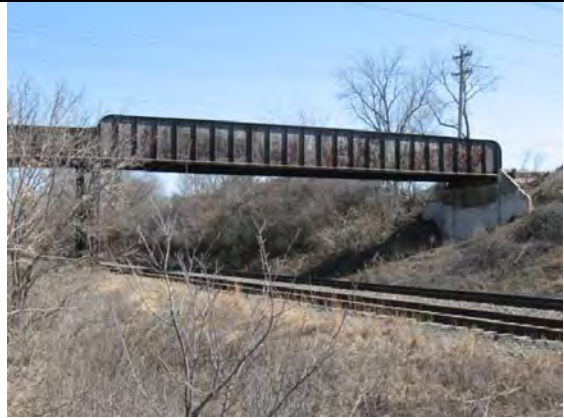
MN&S Bridge, facing SE
