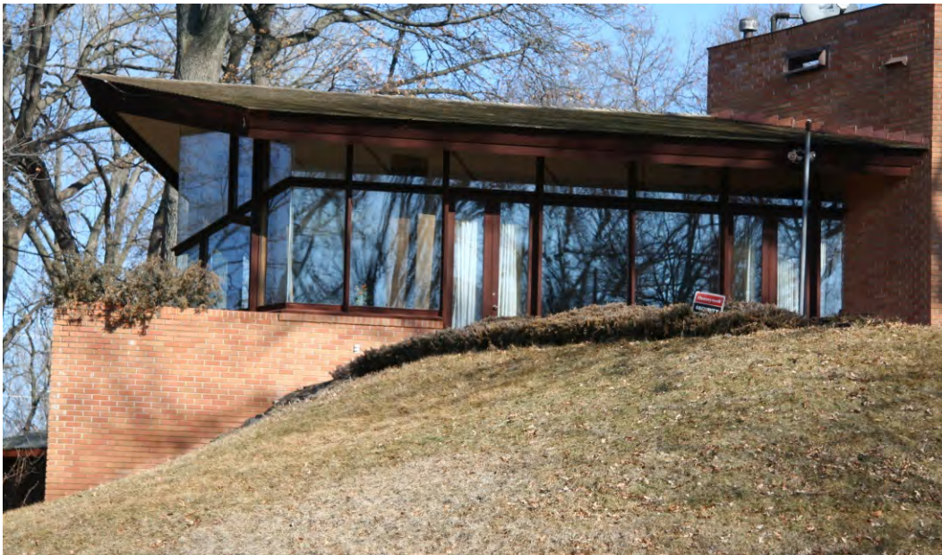
Figure 29. Exterior overview of active area with French doors, bands of windows, and brick planter, view facing east.
