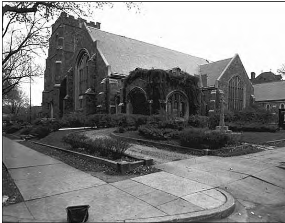
View of the church from the corner of Groveland and LaSalle, with porte-cochere in the center, October 16, 1951 Minneapolis Journal Star Tribune Photograph— Minnesota Historical Society Collections
