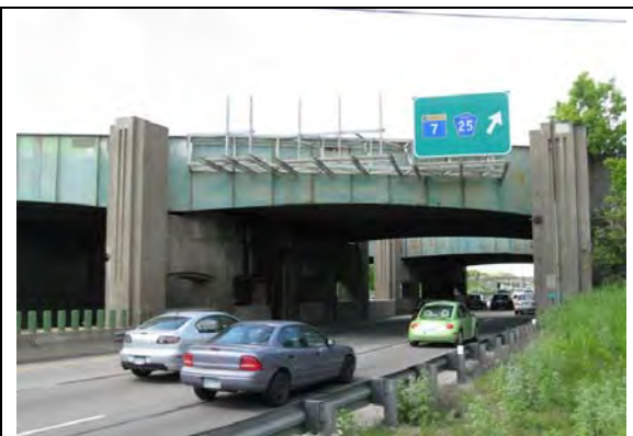
CM&StP Bridge over Hwy 100, facing NW
