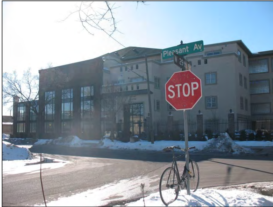
Pleasant Avenue South (east) facade of Western Allied Steel Building. The historic portion of the building is visible at the left. View to southwest.
