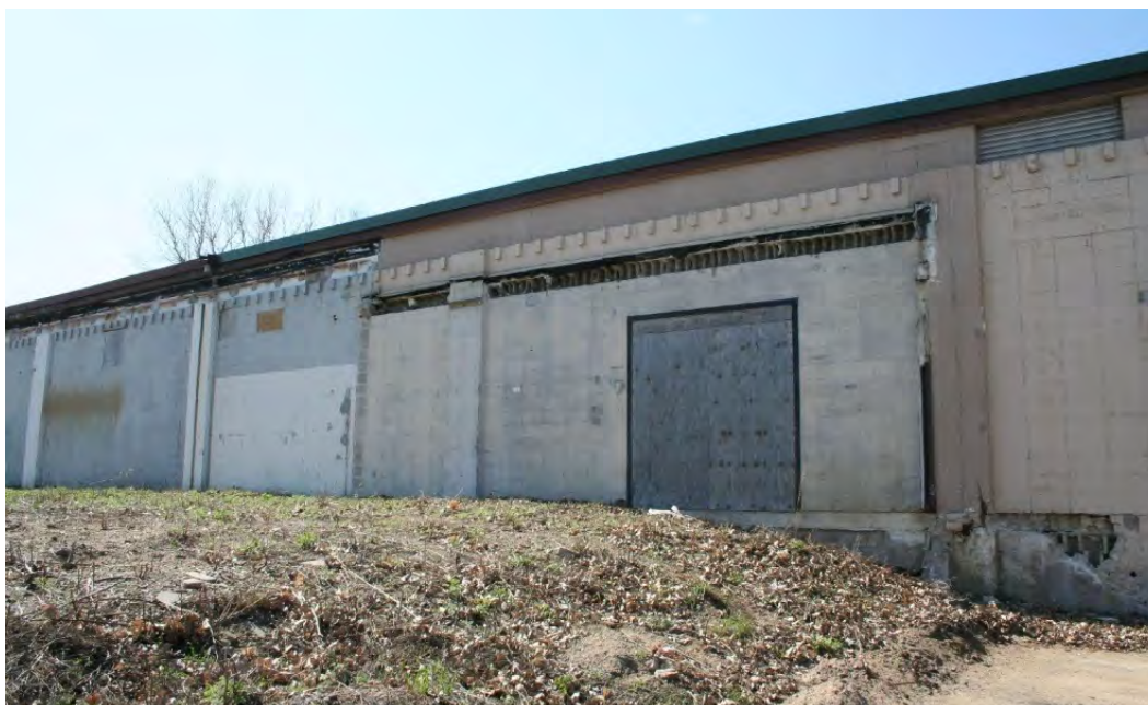
Figure 49. Original loading dock entrance into the warehouse, which projected from the northeast (side) elevation, view facing west.
