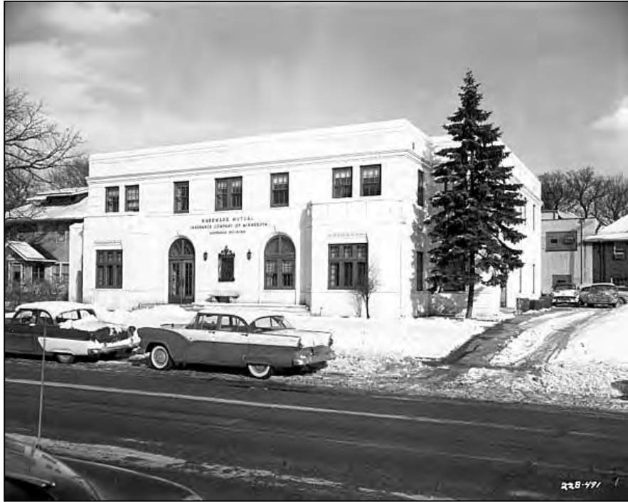
Lee Mortuary in use as a “Research Building” by Hardware Mutual Insurance Company of Minnesota, 1955 Norton and Peel Photograph—Minnesota Historical Society Collections
