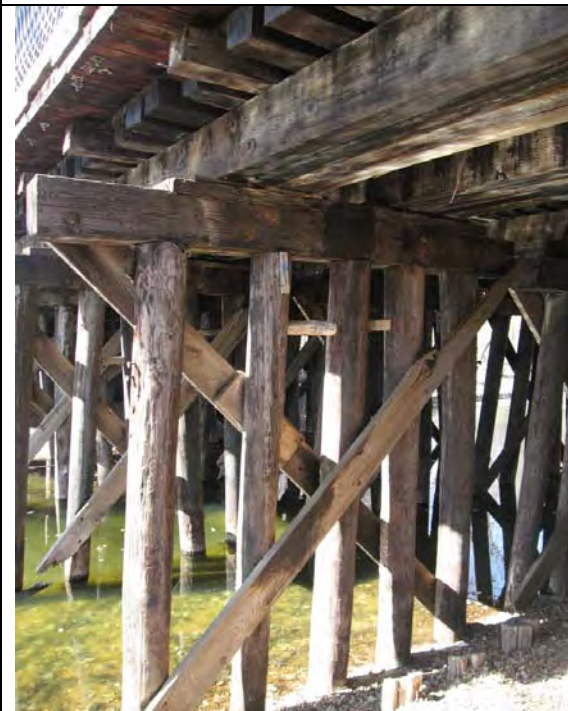
M&StL Bridge over Kenilworth Canal, detail of timber piles
