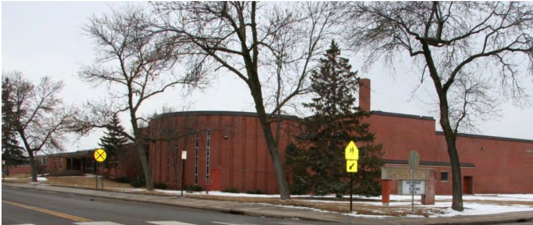
Figure 12. Rounded northeast corner of the core section (1956) of St. Louis Park High School, view facing southwest.
