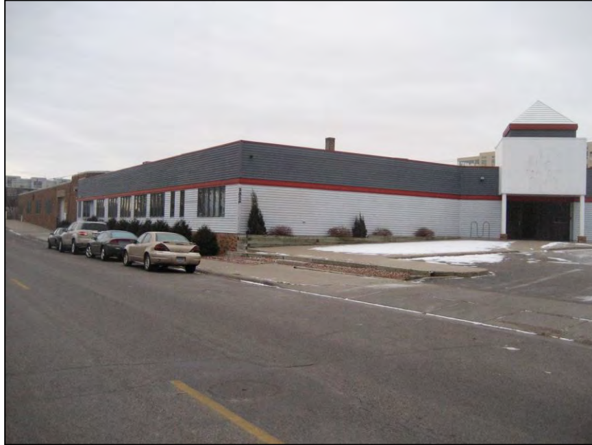
West and north facades of Norris Creameries with historic portion visible at rear. View to south.
