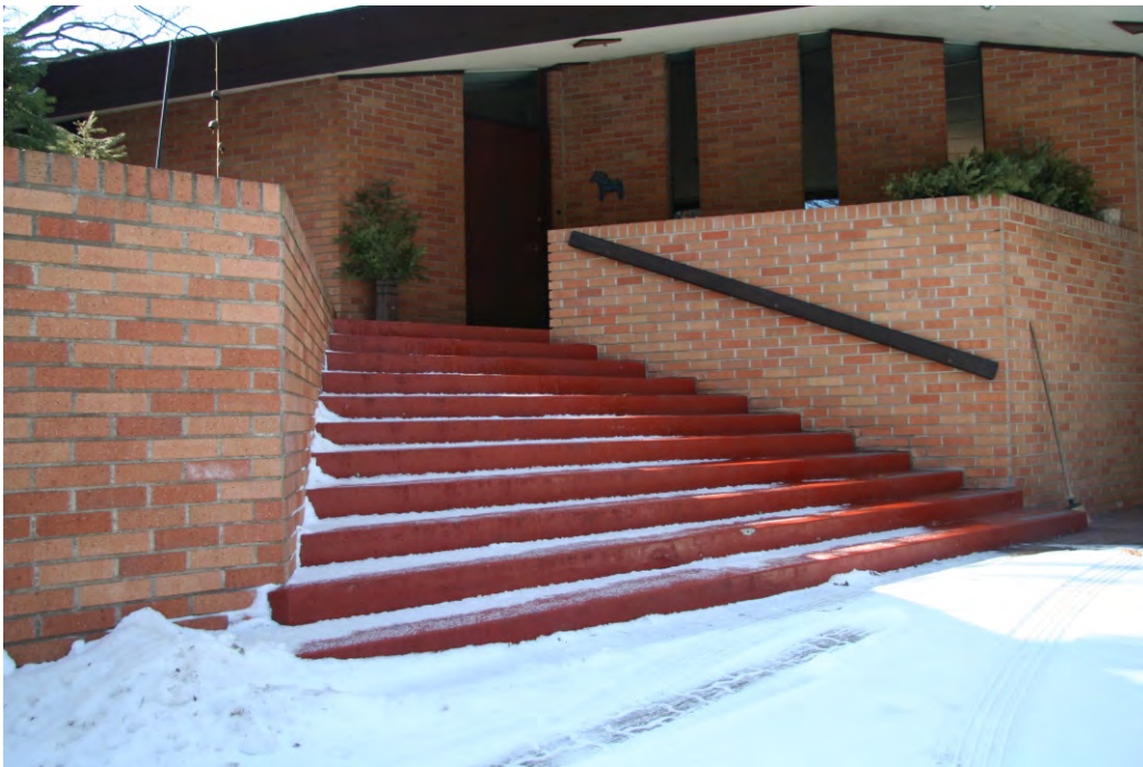
Figure 25. Entryway and stairs, view facing south.
