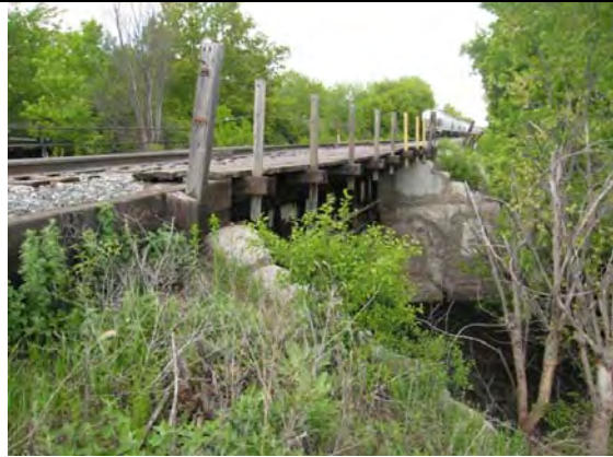
CM&StP Bridge over Minnehaha Creek, facing NE
