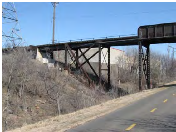
MN&S Bridge, facing NE
