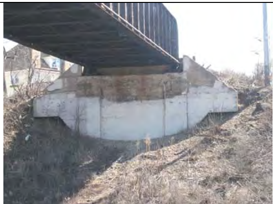
MN&S Bridge, facing S
