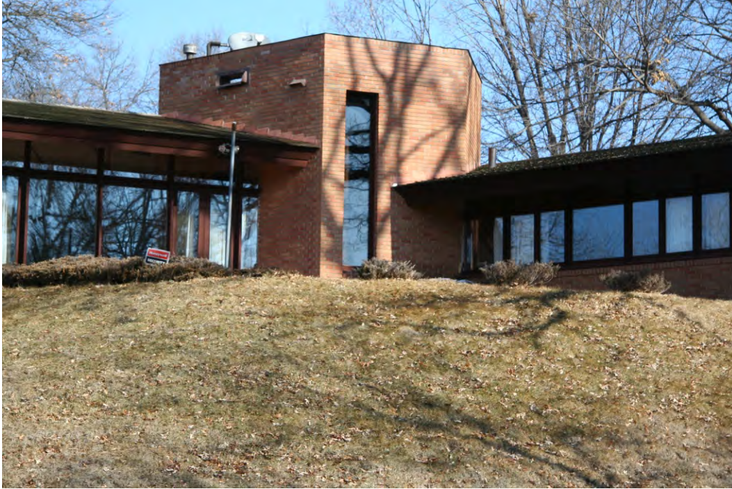
Figure 24. Exterior overview of the kitchen, view facing east.
