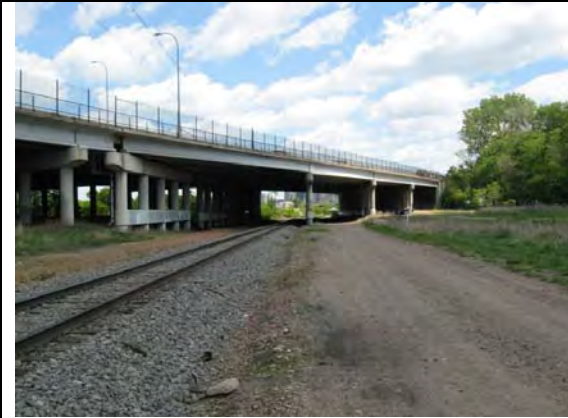
Manitoba/Great Northern Corridor at I-394, facing E
