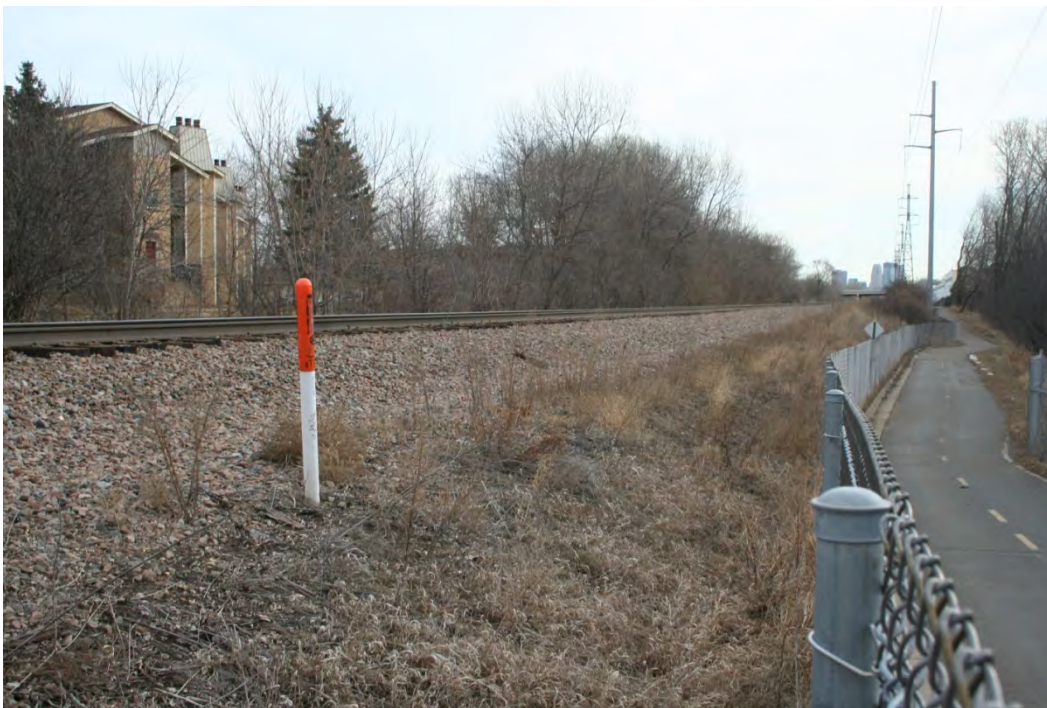
Figure 51. Great Northern Railroad Corridor in St. Louis Park, view facing east toward Highway 100 bridge.
