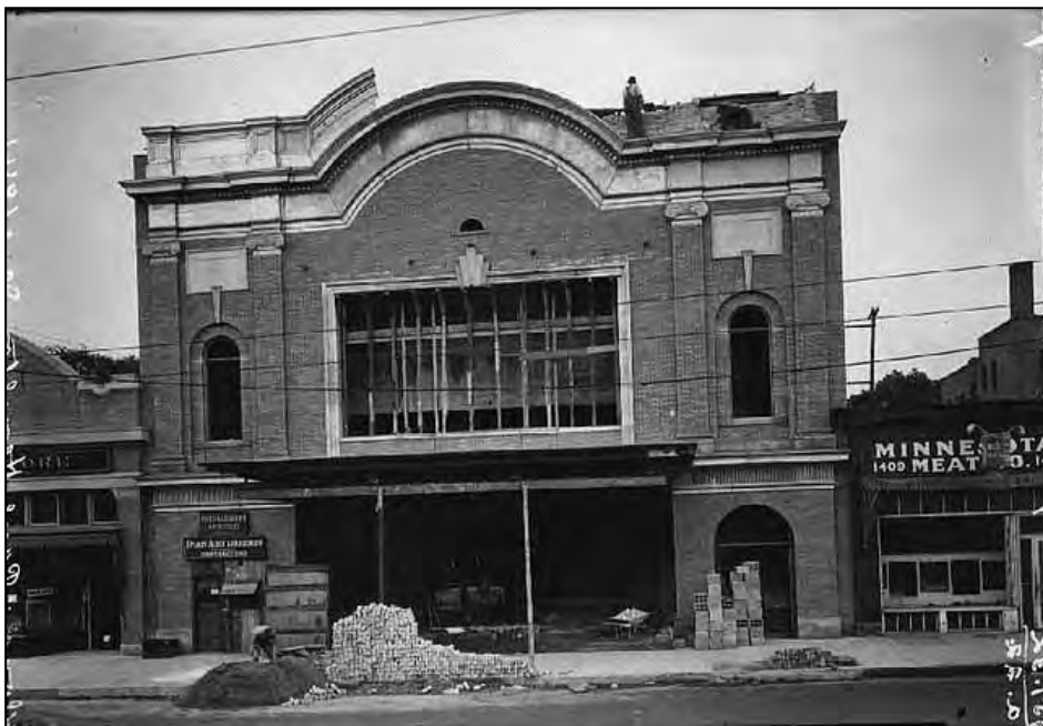
Loring Theater under construction, 1920 Minnesota Historical Society Collections
