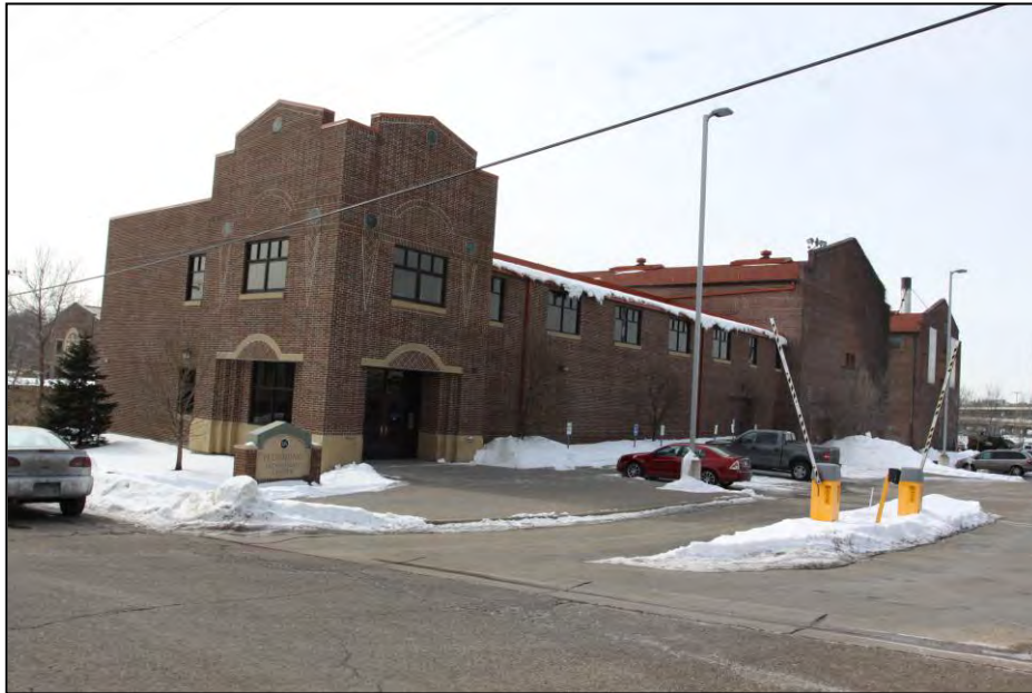
Above: Rear (left) and west facade , looking southeast
