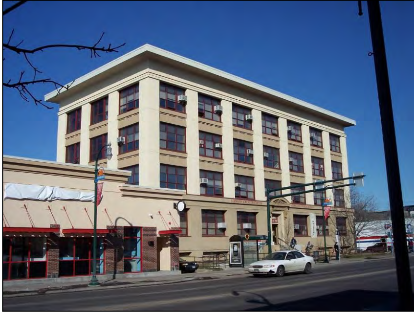
Above: Lake Street facade and west side of original section. View to northeast.
