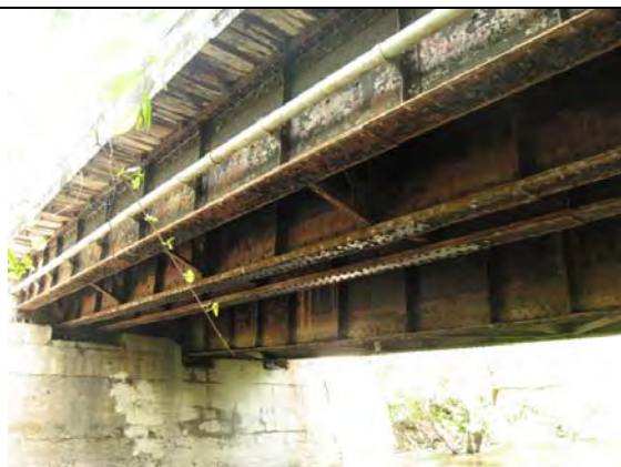
CM&StP Bridge over Minnehaha Creek, facing SE
