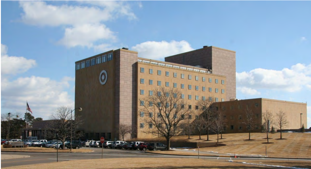
Figure 35. Prudential NCHO, ten-story tower, eight-story north wing, and four-story west wing, view facing southeast.
