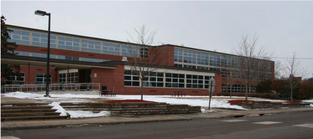
Figure 9. North (West 33 rd Street) elevation of the core section (1956) of St. Louis Park High School, view facing southwest.
