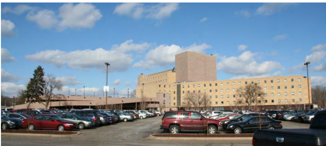
Figure 37. Prudential NCHO, ten-story tower and four-story south wing and parking ramp, view facing north from parking lot.
