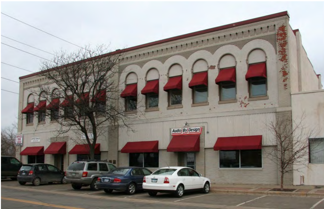
Figure 15. Walker Building, south (front) and east (side) elevations, view facing northwest.
