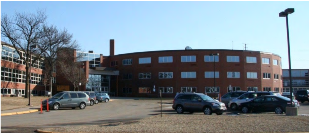
Figure 10. Round wing (1962) of St. Louis Park High School, south entrance (1993) at left, view facing east.
