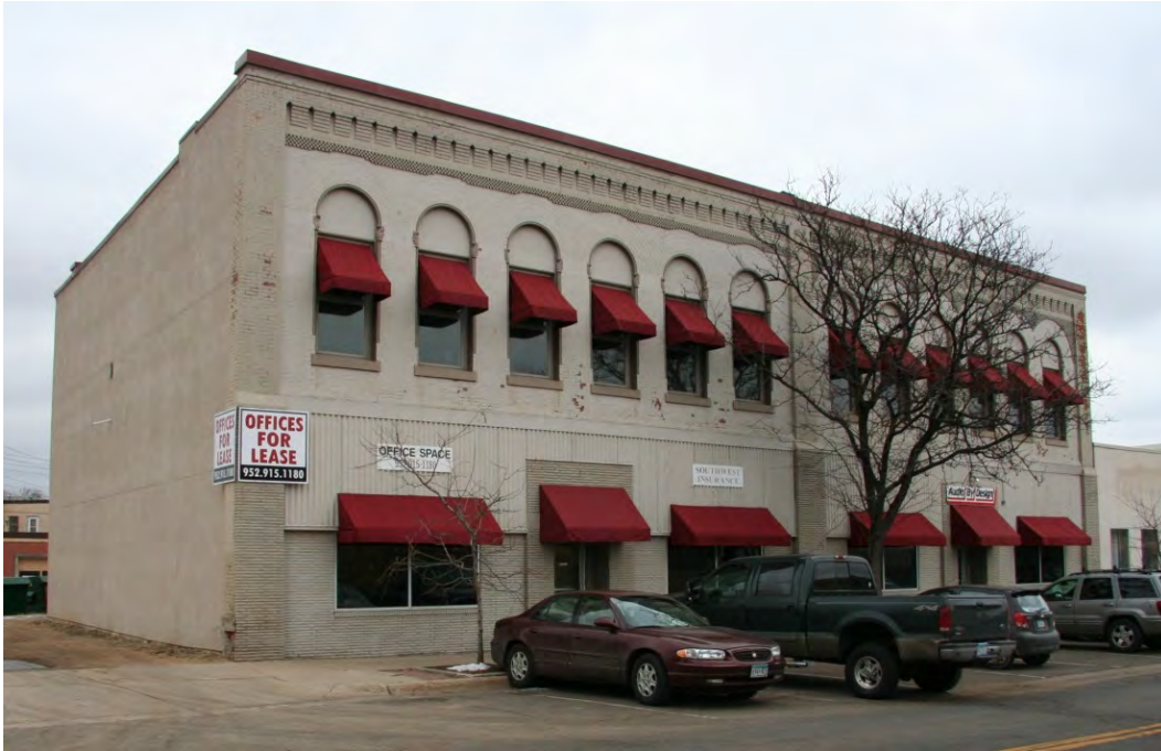
Figure 14. Walker Building, south (front) and west (side) elevations, view facing northeast.
