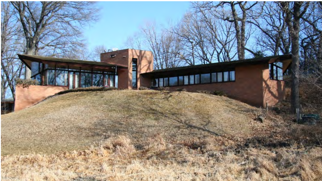
Figure 21. Overview west elevation, view facing east.
