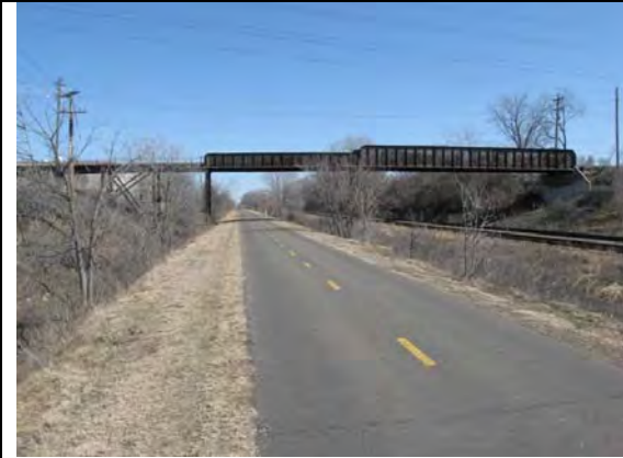
MN&S Bridge, facing E
