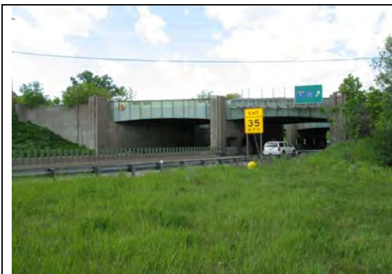
CM&StP Bridge over Hwy 100, facing NW
