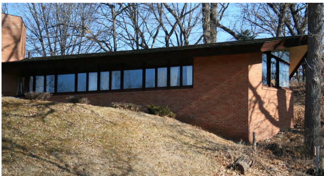
Figure 30. Exterior overview of the quiet wing, view facing east.
