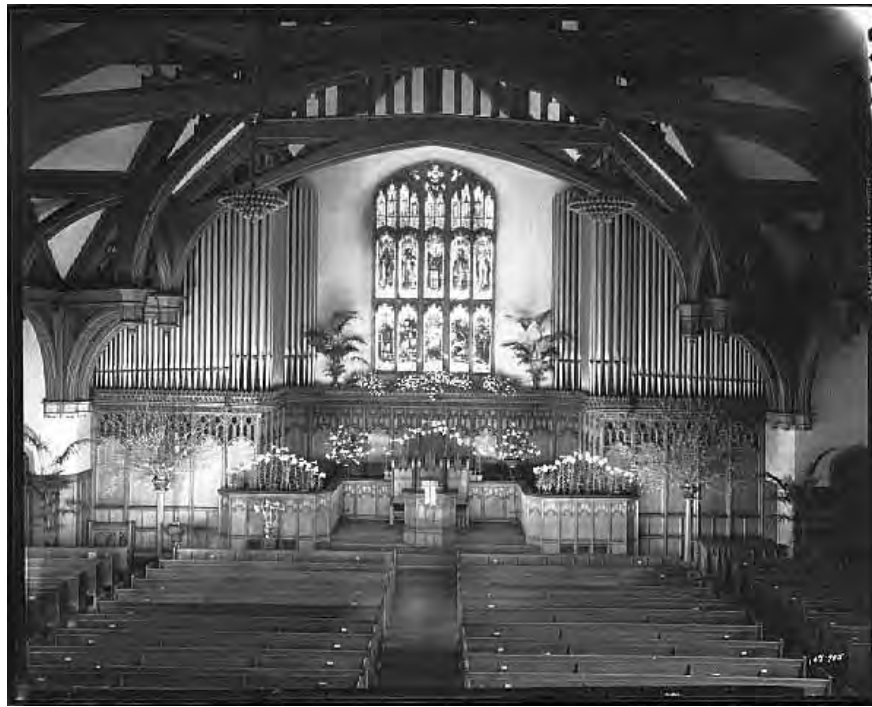
Interior, Plymouth Congregational Church, April 19, 1935 Norton and Peel Photograph—Minnesota Historical Society Collections
