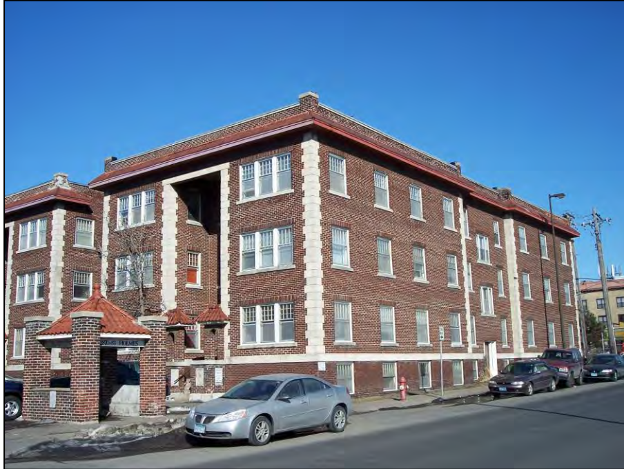
Lagoon Court Apartments, 2883 Holmes Avenue South
