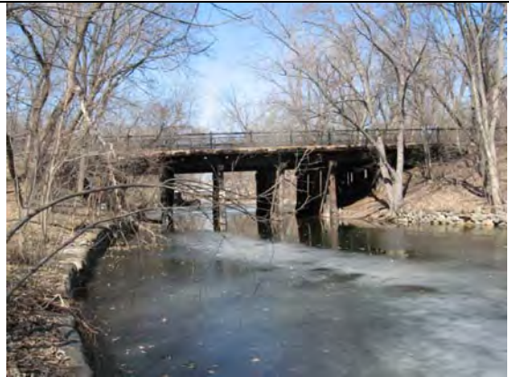
M&StL Bridge over Kenilworth Canal carrying recreational trail, facing NW
