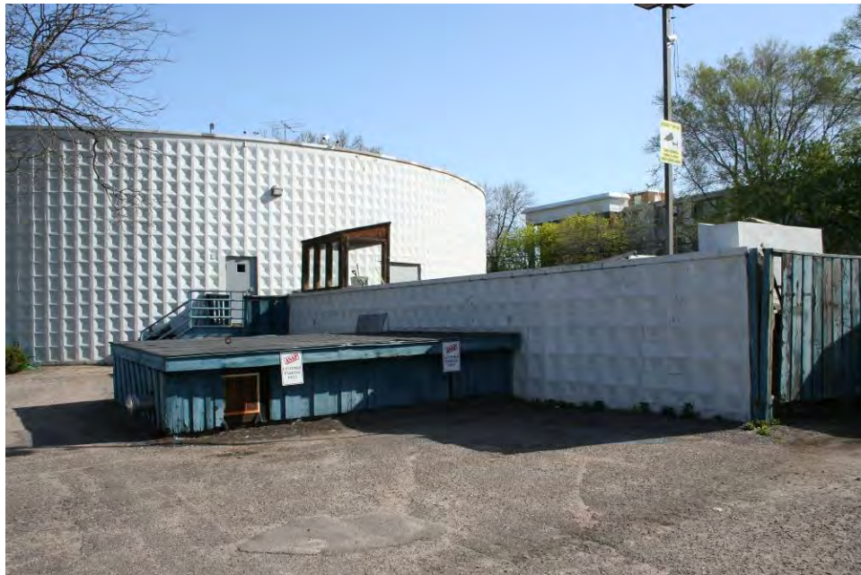
Figure 83. Loading dock on the south portion of the building, view facing southeast.
