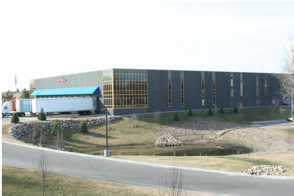
Figure 79. Northeastern elevation of Building #7 showing both glass corners and loading docks, view facing southwest.
