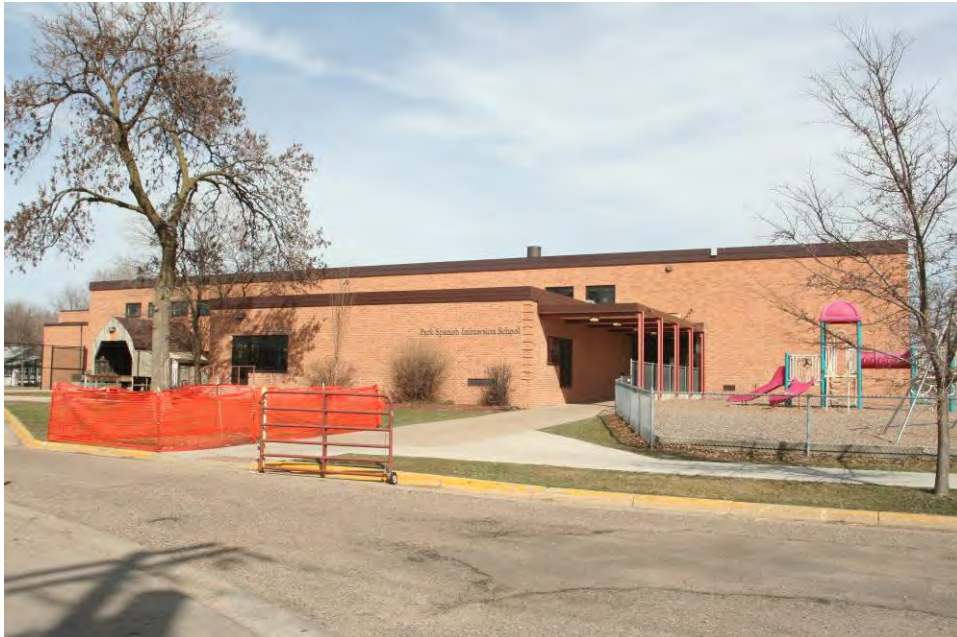
Figure 59. St. Louis Park High School, additions to side (west) elevation, view facing east.
