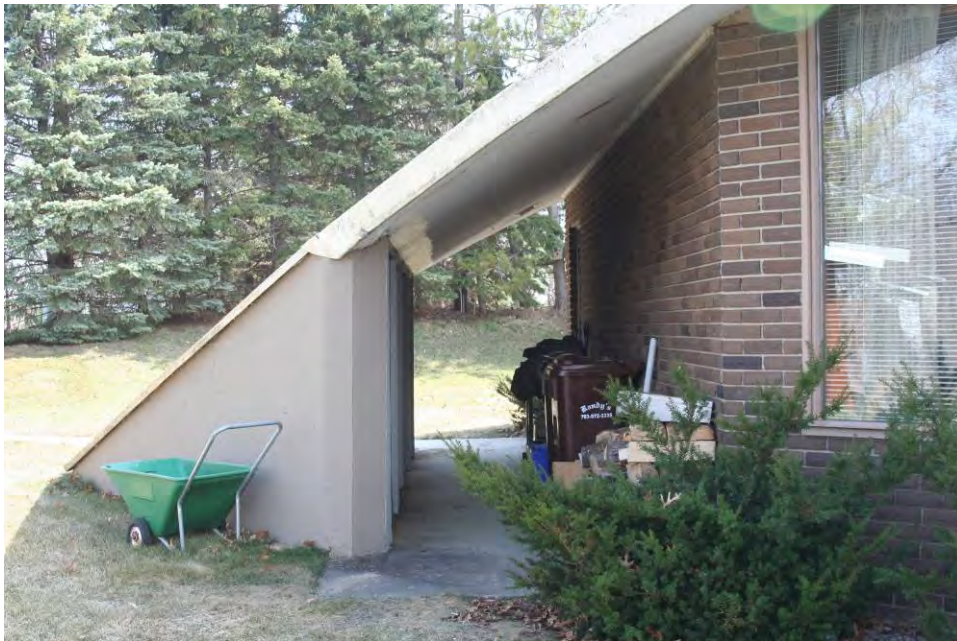
Figure 14. Detail view of the concrete anchors.
