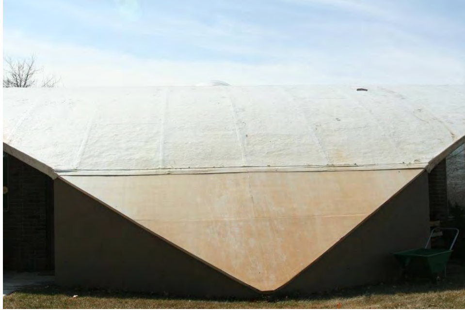
Figure 15. Detail view of the roofing materials.
