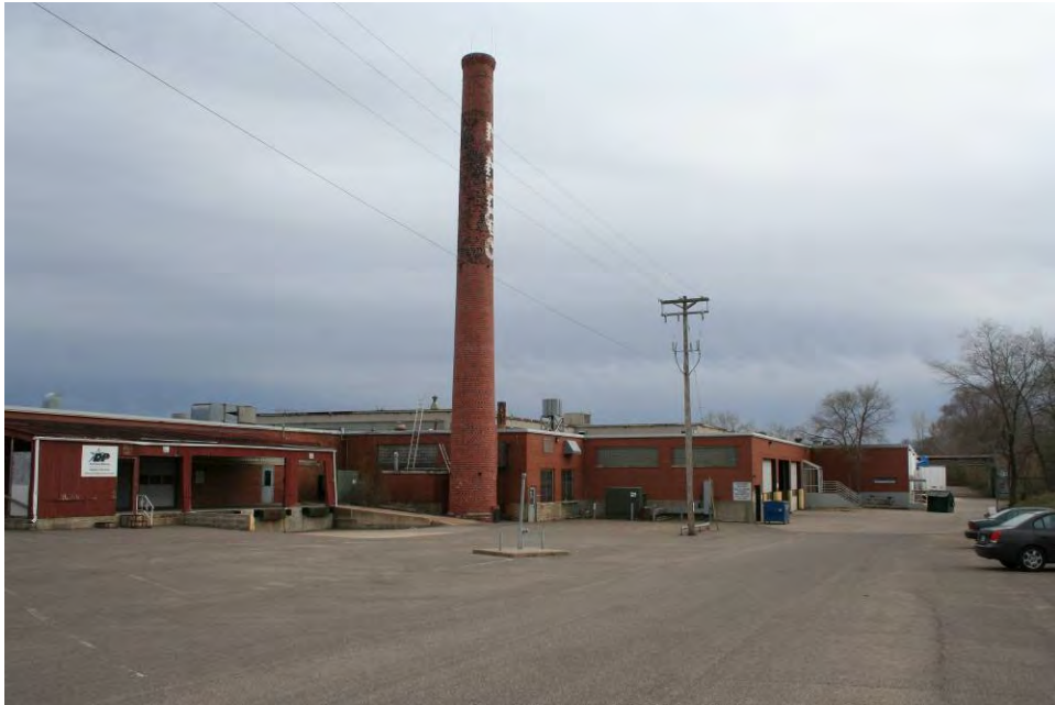
Figure 44. Former Minneapolis Moline building, side (east) elevation, view facing southeast.
