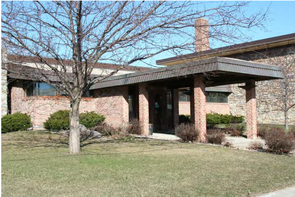
Figure 71. 1984 hyphen addition, front (east) elevation, view facing northwest.
