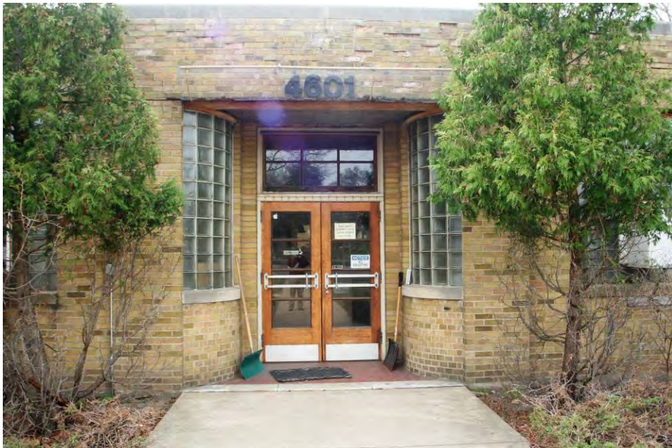
Figure 63. Woodmark Industries Building entrance detail, view facing south.
