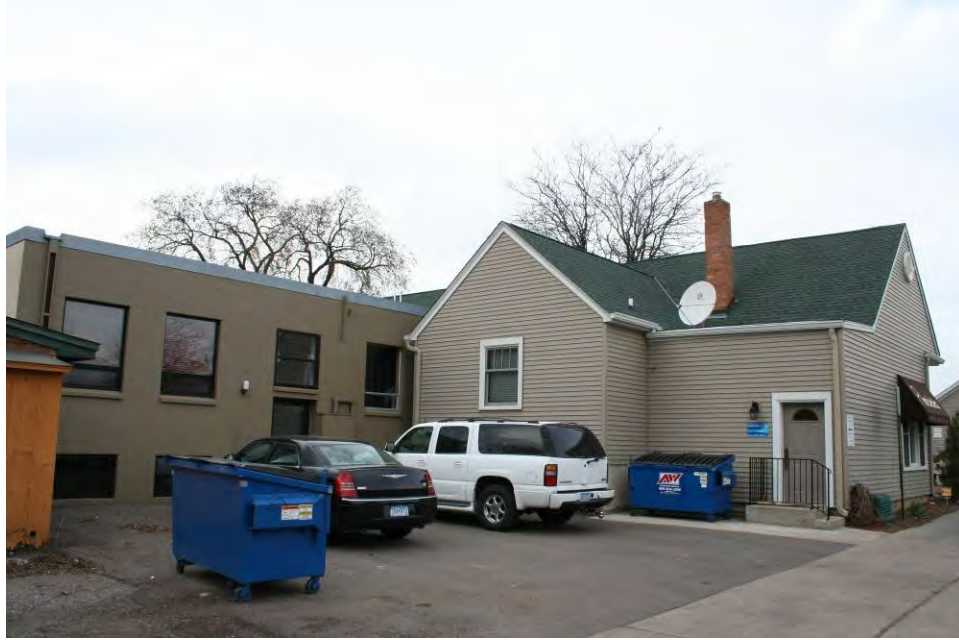
Figure 54. Addition to building immediately north wrapping around east elevation to obscure a portion of the elevation, view facing northwest.
