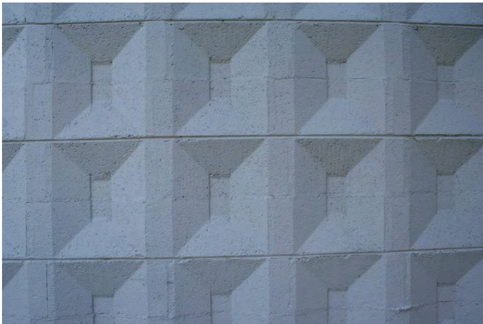
Figure 81. Detail view of the geometric formed concrete pattern.
