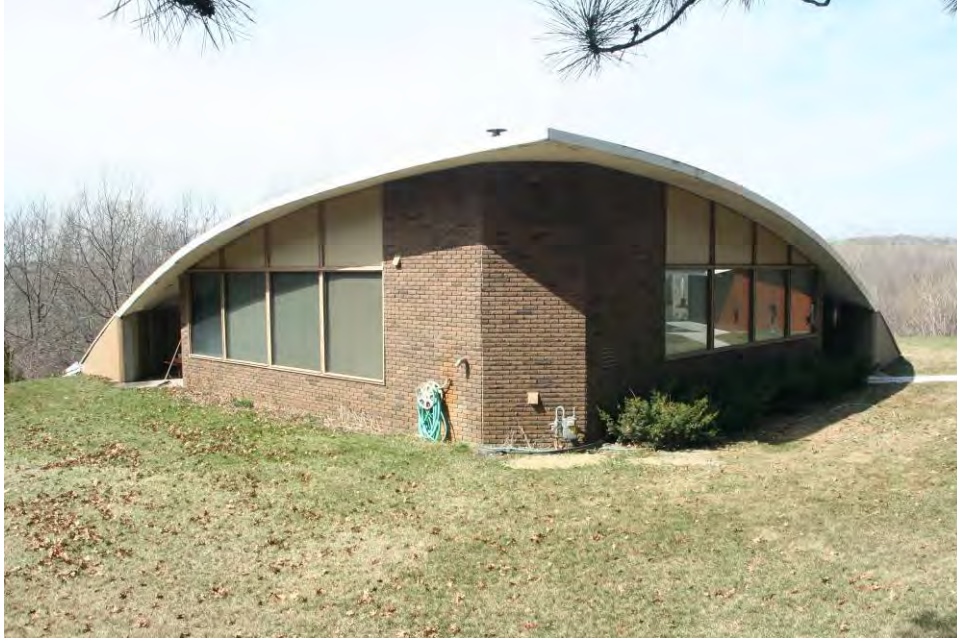
Figure 13. Note how the north and south sides of the roof are pinned to the ground while the east elevation is allowed to extend, view facing southwest.
