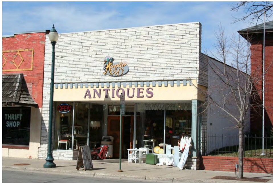
Figure 36. The c.1960 building located at 911 Mainstreet, view facing northwest.
