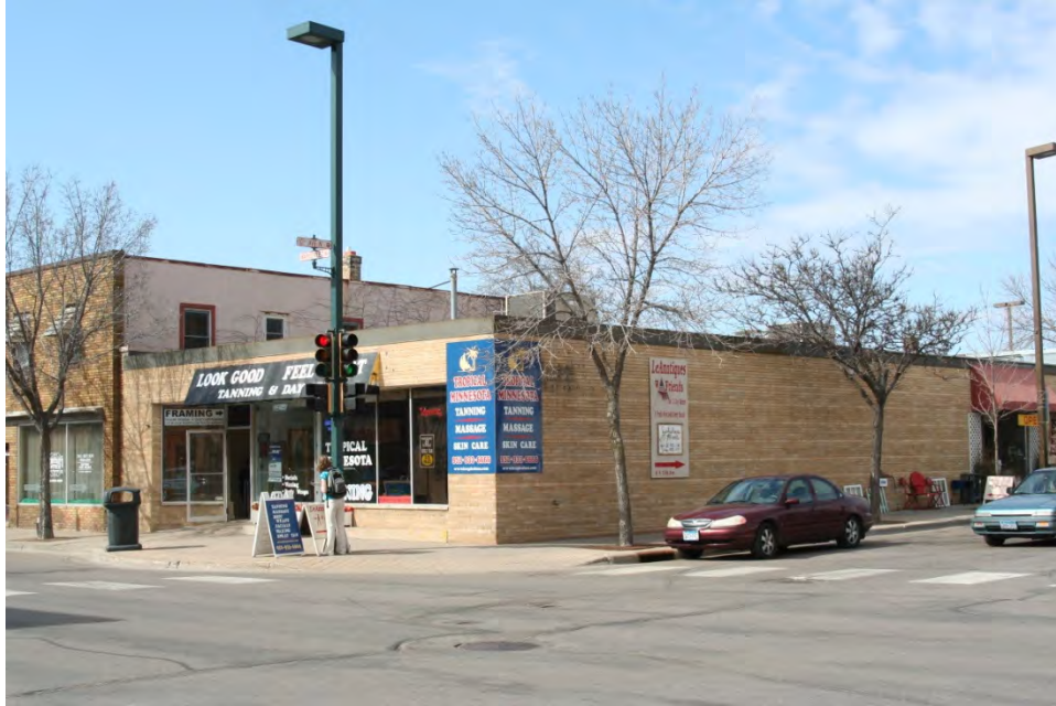
Figure 37. The 1958 Kokesh Hardware Store located at 1001 Mainstreet, view facing northwest.
