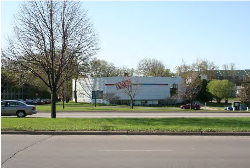
Figure 80. Front of the Motor Travel Lodge Building, view facing south.
