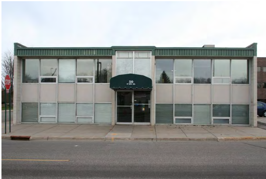
Figure 50. East (primary) facade, view facing west.
