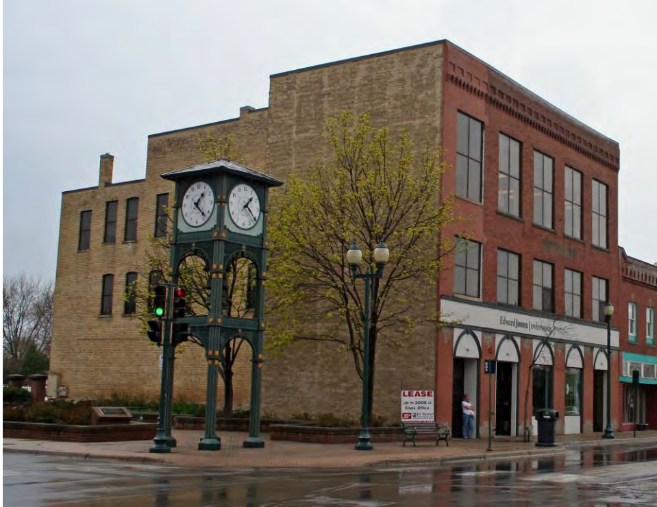
Figure 33. 1902 Olson Building located at 906-908 Mainstreet, view facing southwest.
