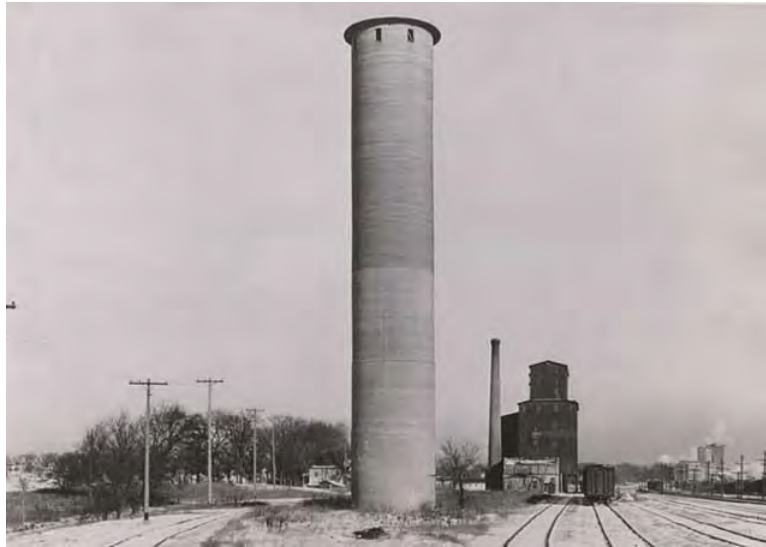
Figure 8. Peavy-Haglin Experimental Concrete Grain Elevator, located along the rail corridor, c.1908 (photo courtesy of the Minnesota Historical Society, Negative 26073).
