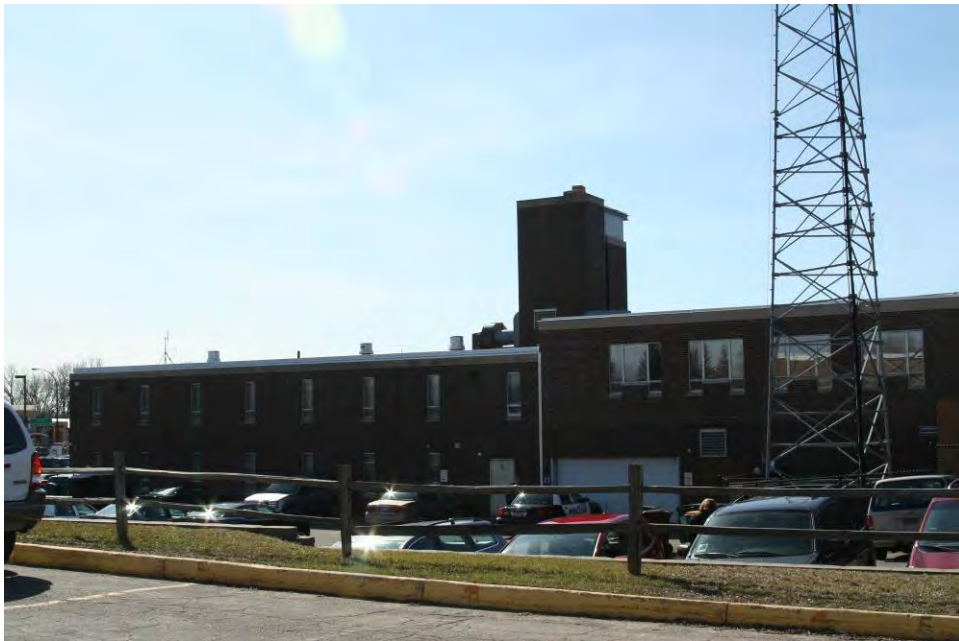
Figure 25. East elevation of Hopkins City Hall, including the hose drying tower, view facing southwest.
