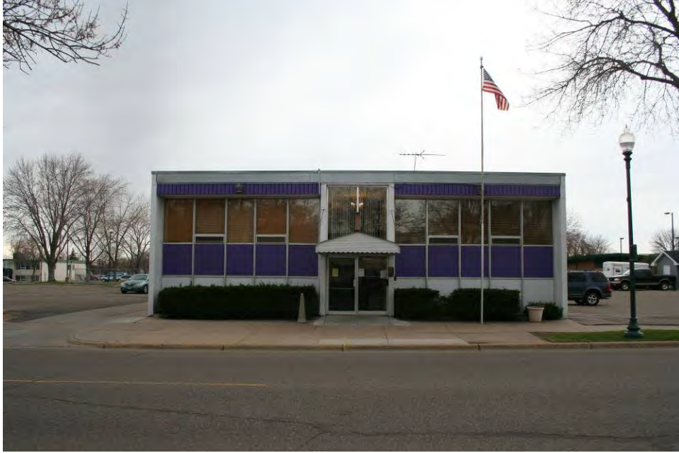
Figure 47. East facade of 30 8th Avenue South, view facing west.
