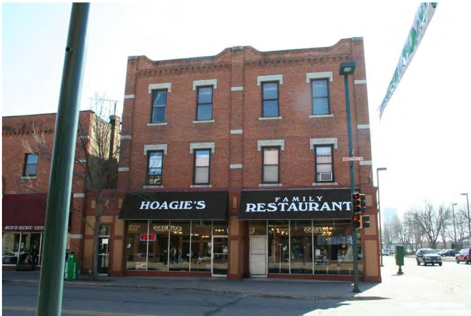
Figure 32. 1893 Olson Building located at 824 Mainstreet, view facing south.
