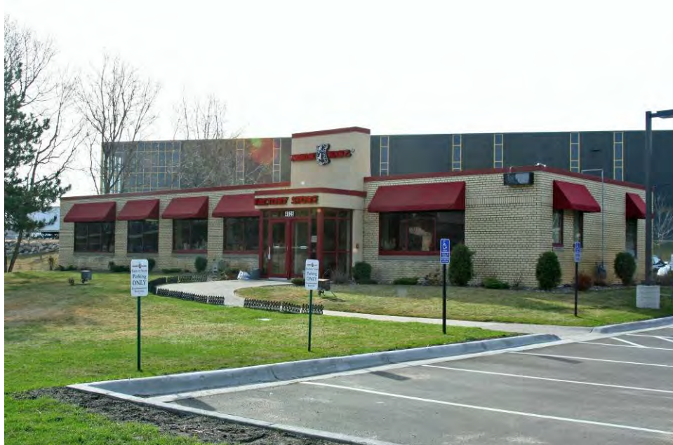
Figure 77. Building #4 facade and west elevation, the structure was built in 1950 and added to the Northland Aluminum building inventory in 2006, view facing southeast.
