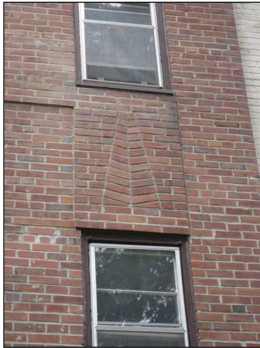
Detail of brickwork on apartment buildings
