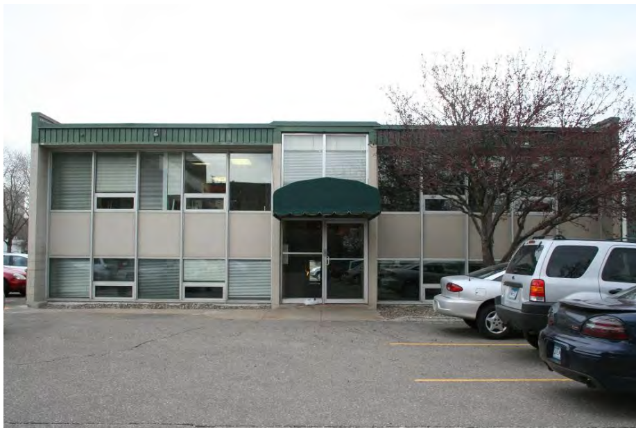
Figure 52. West elevation, view facing east.
