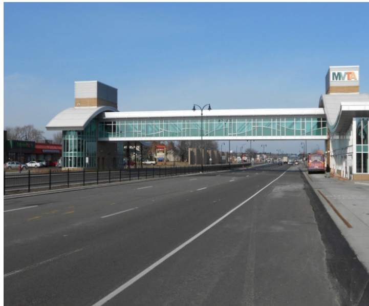
Figure 8: Apple Valley Transit Station located on recently completed bus shoulder project
