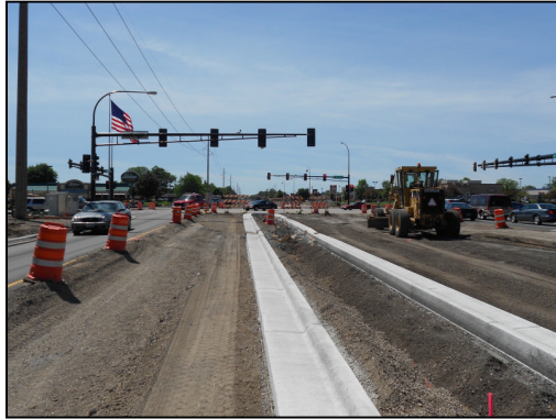
Figure 9: Construction along County Road 42, before and after
