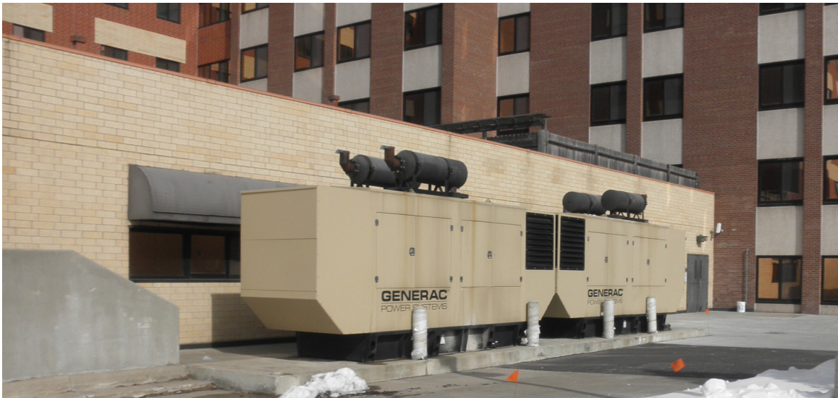
A typical diesel generator installation at a nursing home located near resident rooms. Low smokestacks result in poor air dispersion, and people can be exposed to exhaust through windows and building air intake vents.
