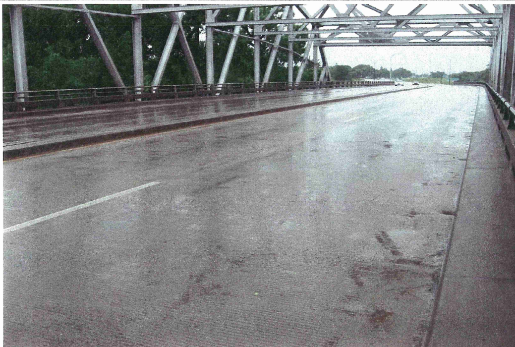
Photo 3 – General view of top of deck, looking east.
