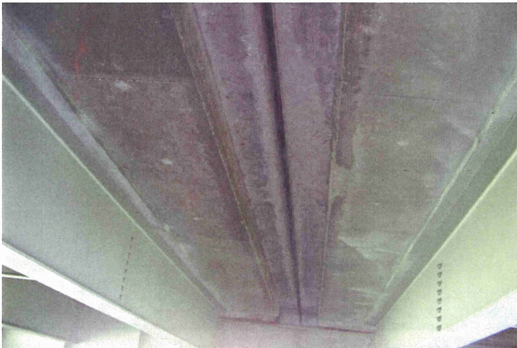
Photo 6 – Typical condition of longitudinal deck joint along center line of structure. Looking west.
