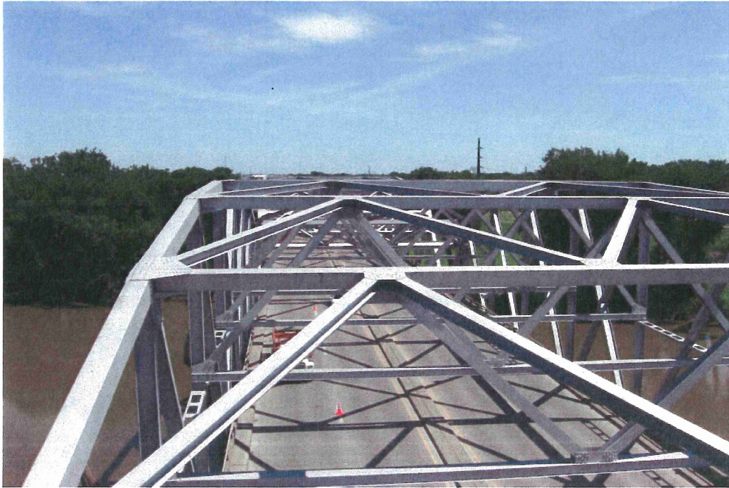
Photo 9 – General view of upper chord members, looking east.
