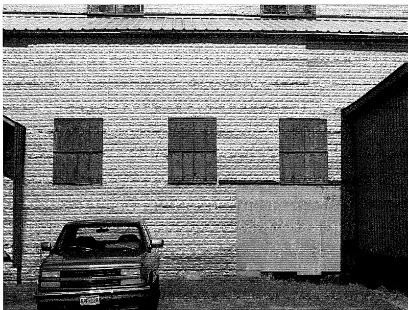
Figure 41. SL-VGC-150, looking north at detail of metal cladding on south elevation, 11/10/11.
