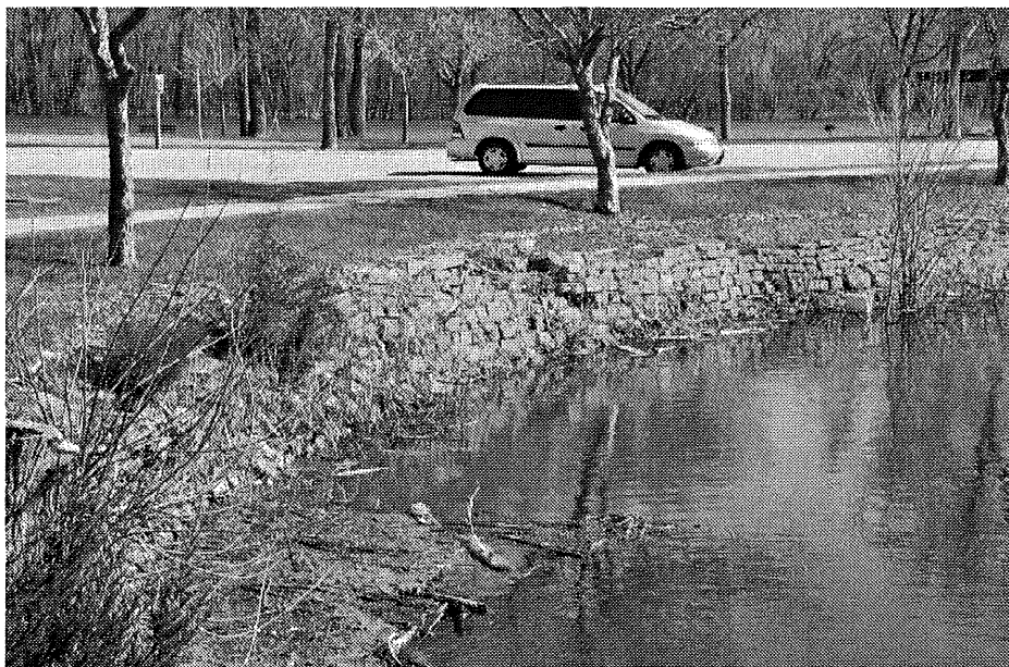
Fig. 26. Levee Rd. Red Wing Harbor and Levee, retaining wall of dry laid salvaged concrete on the north edge of Vogel Harbor (facing N)
