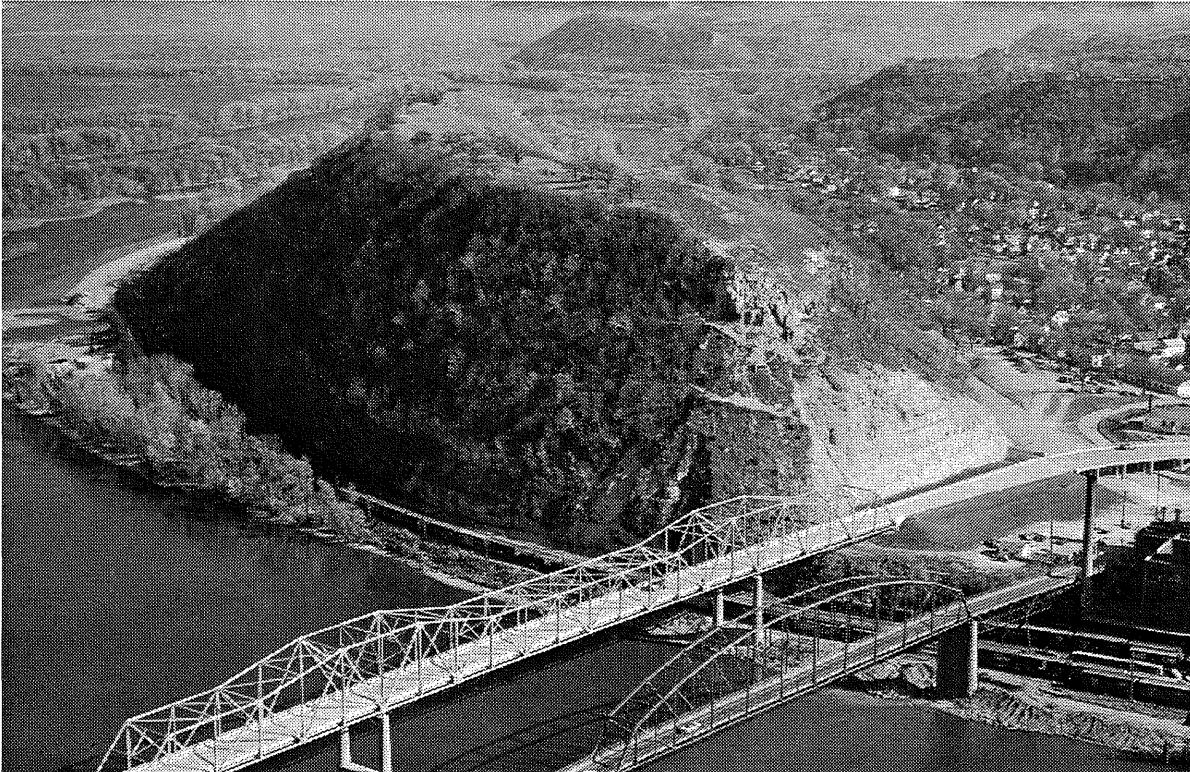
Fig. 3. Newly-completed Bridge 9040 and its 1895 predecessor; note that the western end of Barn Bluff was shaved off for the new bridge approach; October 1960, photo by St. Paul Dispatch (Minn Hist Soc) (facing E)
