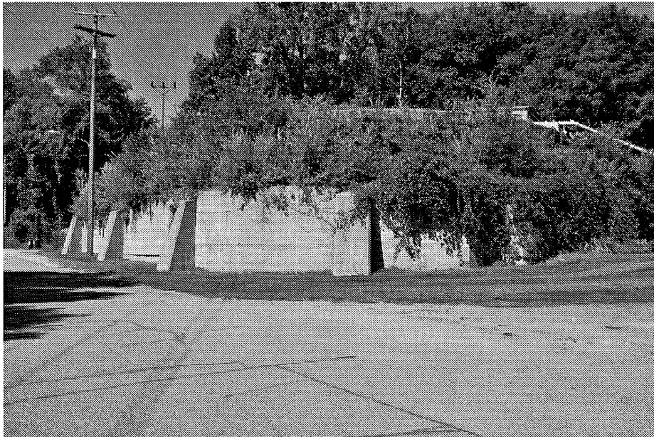
Fig. 172. ca. 700 5th St. E. Red Wing Water Dept. Pump House 2, buttressed concrete storage reservoir (facing W)
