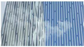
Patterns on the outside of glass, such as that shown above, are more effective than patterns on an inside surface. Photo: Hans Schmid
