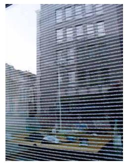
The glass facade of SUVA Haus in Basel, Switzerland, renovated by Herzog and de Meuron, is screen-printed on the outside with the name of the company owning the building. Photo: Miguel Marqués Ferrer
