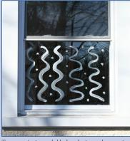
Tempera paint is a washable, long-lasting, and non-toxi solution to preventing bird/window collisions.
