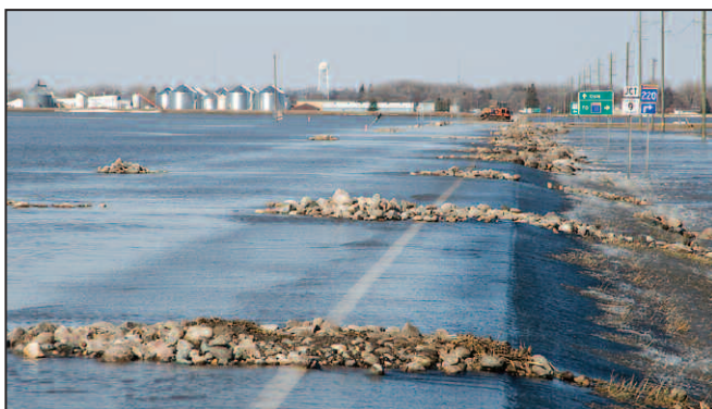
April 9, 2009 – This unusual mitigation method employs large stones to divert and break up water from the Red River as it flows over and under a road surface near Oslo, Minn. The SEOC was activated for four weeks during Red River floods in 2009. Photo: Mike Moore, FEMA
