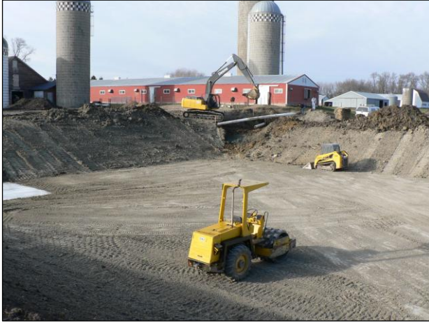
Figure 1. Typical manure storage pit under construction in Stearns County
