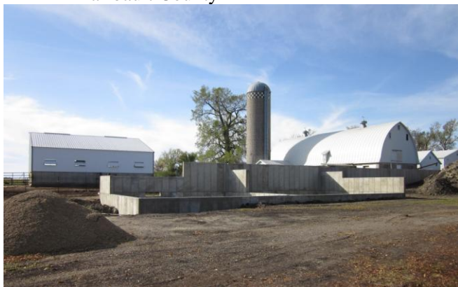
Figure 27. Ramped manure pit on Gary Yokiell Farm, Faribault County
