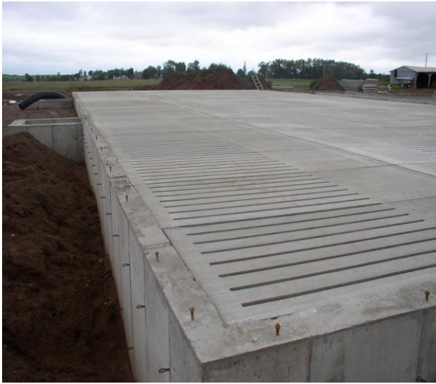
Figure 3. Typical concrete slatted floor manure storage basin
