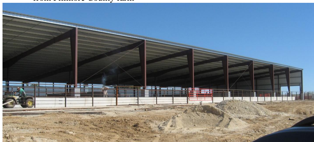
Figure 28. Mono-slope total confinement roof structure that controls feedlot runoff from Fillmore County farm
