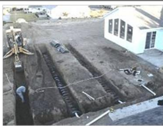
Figure 11. Typical septic system installation
