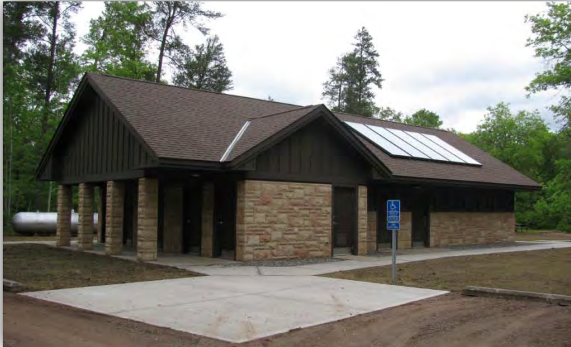
Sanitation building with solar thermal system at St. Croix State Park
