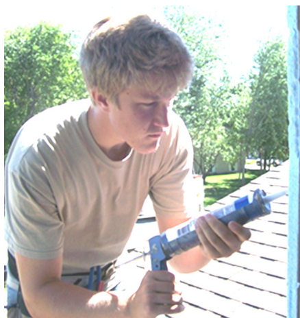
Ryan applies caulk to a window frame of a new Habitat for Humanity house.
