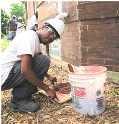
Derek mixing mortar for his tuck-pointing project.
