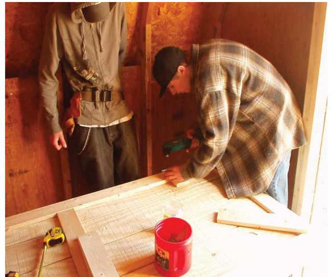
Photo above: Youthbuilders measuring strips of wood for storage shed.
