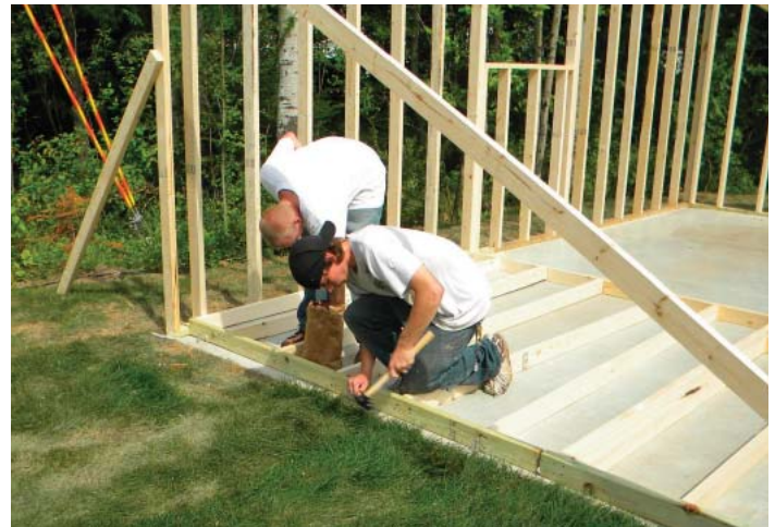
Above photo: Nick and Ricky working on side frame
