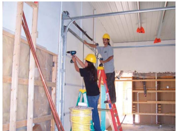
Photo above: Bobby and Cheyenne are attaching a garage door to a single family low-income home for a Red Lake tribal family.
