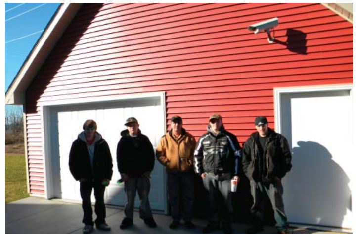
Photo above: Youthbuild crew next to newly constructed Foyer Storage Facility
