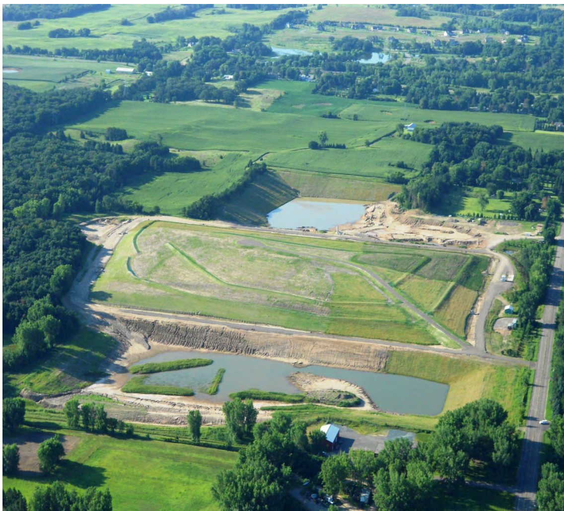
Aerial view of nearly completed construction at the Washington County Landfill
