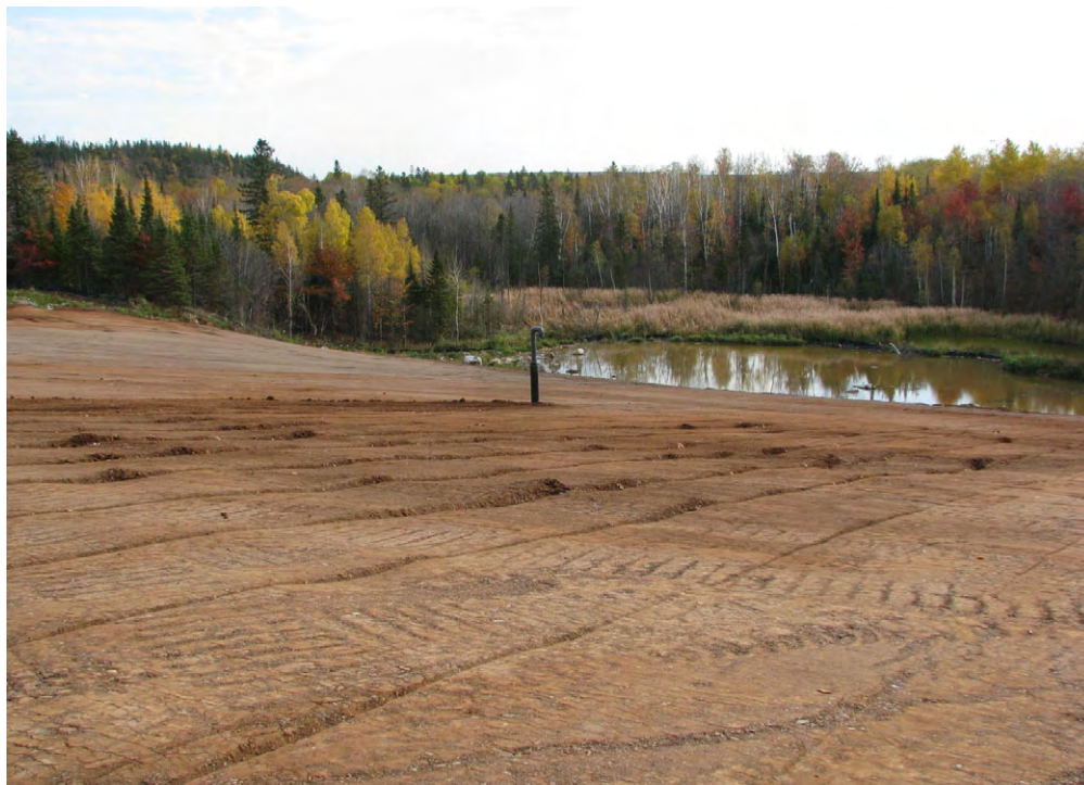
Cover construction at the East Mesaba Landfill, St. Louis County
