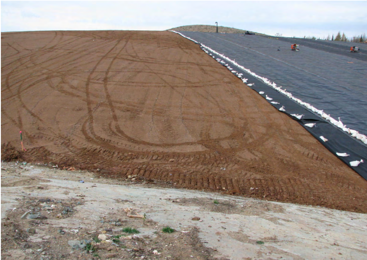
Laying synthetic cover over drainage layer at the East Mesaba Landfill, St. Louis County
