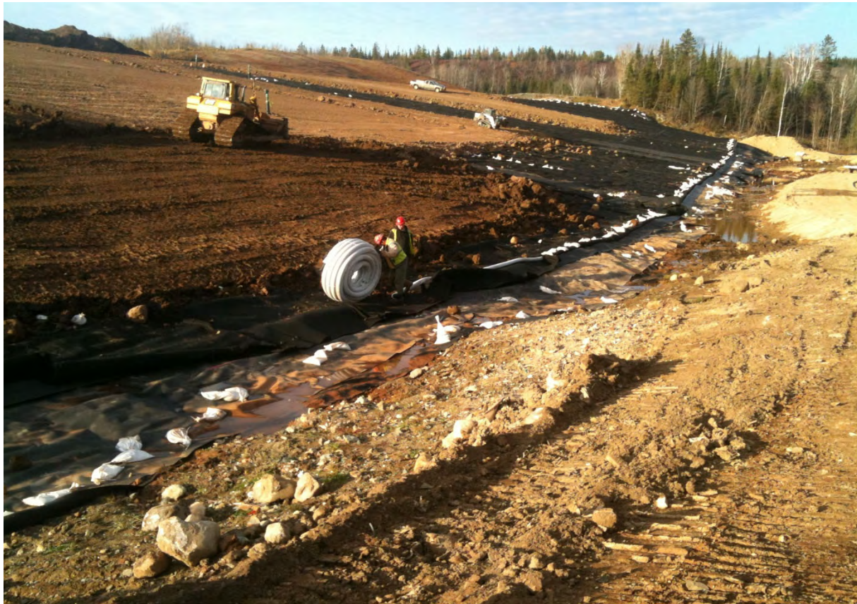
Cover construction and installation of toe drain at the East Mesaba Landfill, St. Louis County
