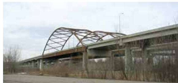
Report 2010-39, “ Development of an Advanced Structural Monitoring System for Fracture Critical Steel Bridges, ” studied tiered-arch bridges like the Cedar Avenue Bridge. These bridges lack redundancy: The failure of a structural member could lead to collapse. They are consequently particularly important to monitor.
