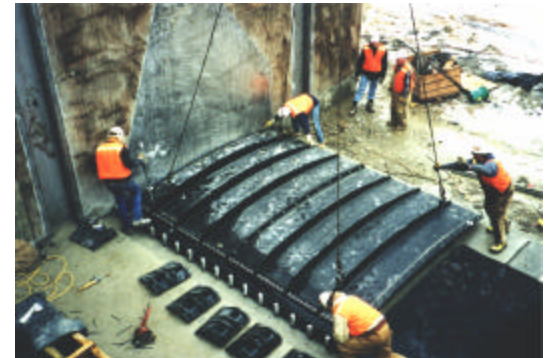
Installation of Gate Panels
