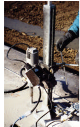
Drilling of Anchor Bolt Holes
