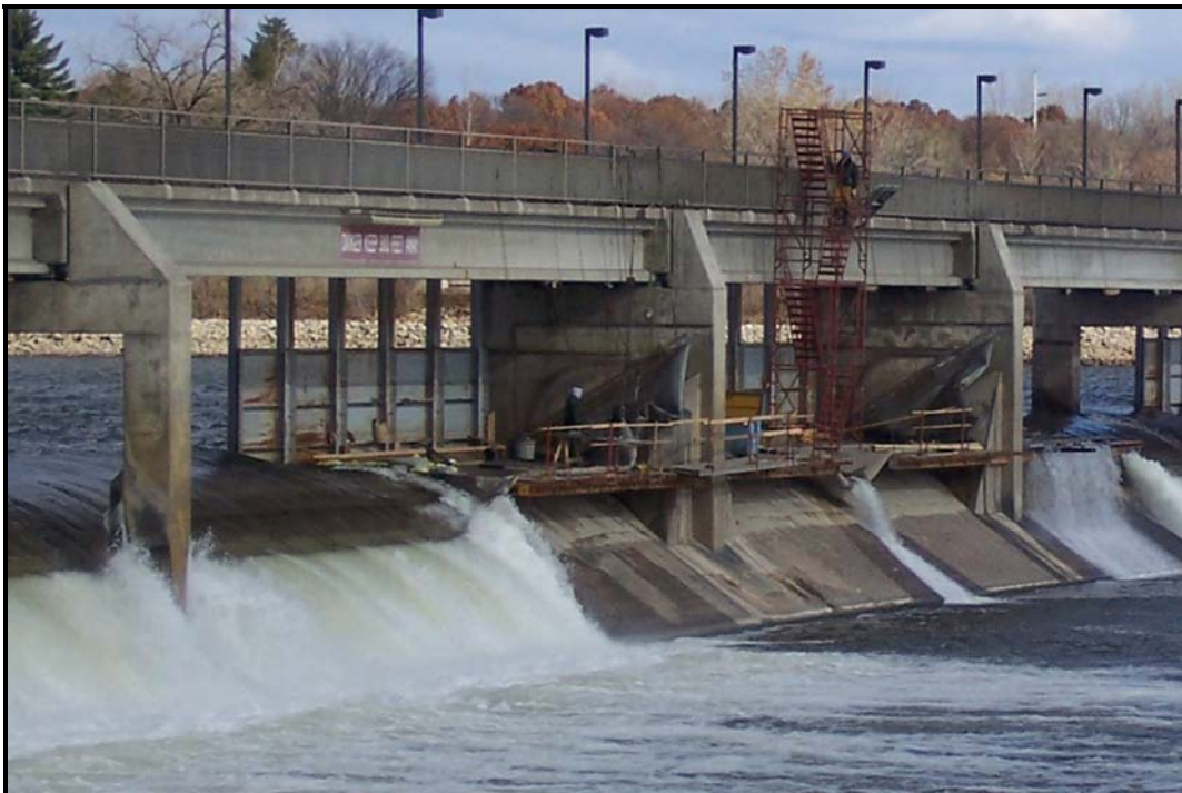
Photograph 21 Inflatable Gate Repair Operation
