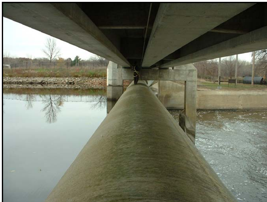
Photograph 3 Main Spillway Inflatable Gate, Bridge Girders, and Bridge Pier
