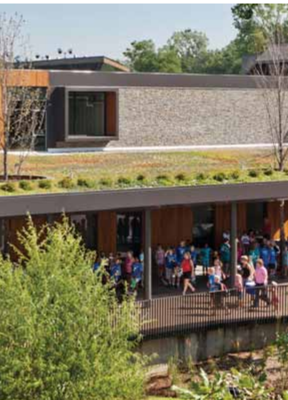
Top | The old whale tank was reborn as the Target® Learning Center. Bottom | An 11,000 square foot vegetative roof creates habitat for wildlife while reducing storm water runoff.
