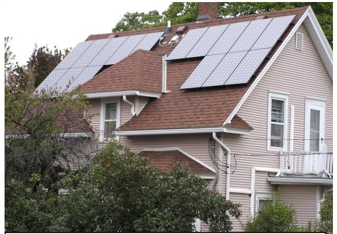
Crystalline silicon panels on a Saint Paul home.
