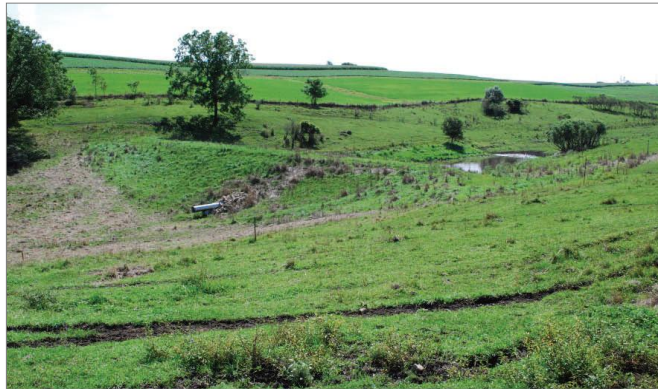
Figure 12. Water and Sediment Control Basin, Southeast MN
