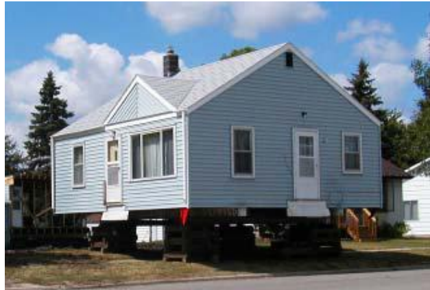
Figure 8. House Relocation from Floodplain
