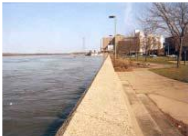
Figure 10. Floodwall at Winona, MN
