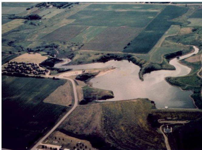
Figure 15. Lake Laura Flood Reduction Impoundment, Redwood County
