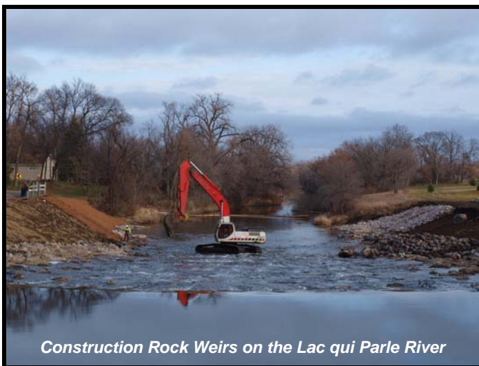
Construction Rock Weirs on the Lac qui Parle River
