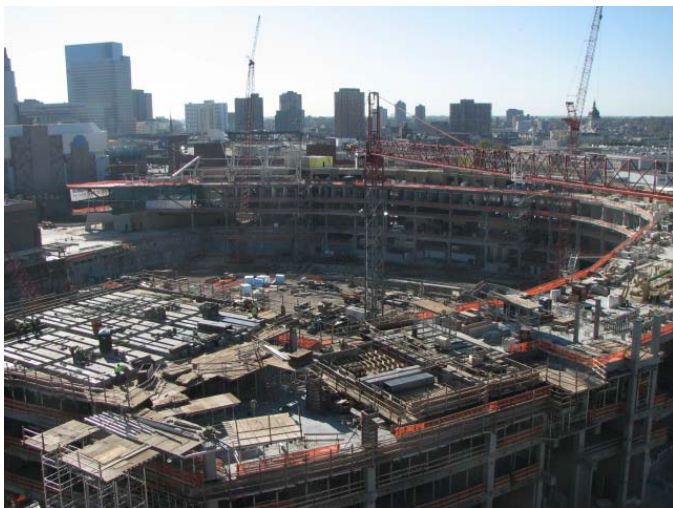
Target Field underway
