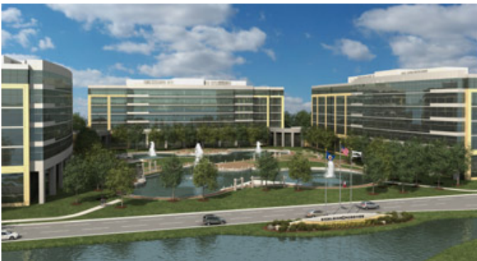
Excelsior Crossings, Hopkins. Before: vacant Supervalu warehouse. After: Artist's rendering of 3-building project when complete.
