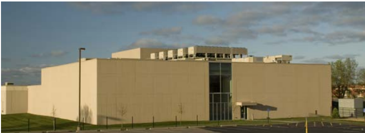
New 40,000 sq. ft. R & D facility in Plymouth, for McQuay Inc: advanced HVAC technologies testing. Submitted for silver LEED certification, achieving 75 percent energy recovery diverted back into the system as well as water-efficient landscaping, recycled construction waste, low-emitting sealants and locally purchased materials. Photo by permission of McQuay International.
