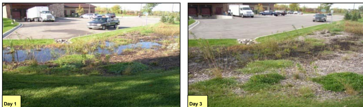
Figure 6.3 Lakeville Municipal Liquor Store, 160 th St. and Galaxie Ave. Pictures were taken October 7 - 9, 2009, after receiving 3.79 inches of rain from October 1-6. This site did not always dry completely, was found to have floodwater mosquito larvae, and might be able to support mosquito larval development to adult emergence if rainfall was sufficient. Two other rain gardens constructed on the same property never held standing water at any time they were inspected in 2009.
