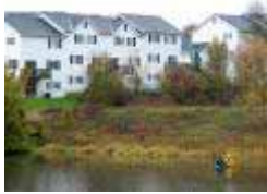
A storm water pond in Woodbury
