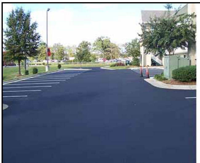
Figure 7. Sealcoat products are applied to parking lots and driveways in an effort to protect the asphalt pavement and for cosmetic purposes (image from: http://www.autocyclesealcoating.com/wp-content/uploads/2008/07/sealcoat3.jpg ).
