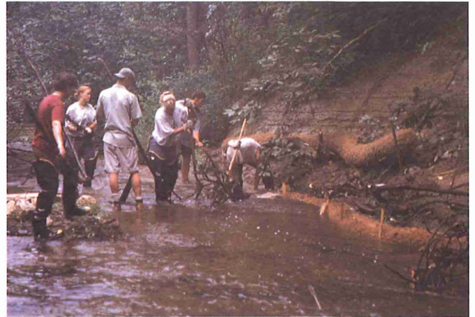
Citizens stabilize eroding stream banks at Brown's Creek. Bank restoration helps prevent sediment and sand from settling in the stream bed, resulting in better trout reproduction.
