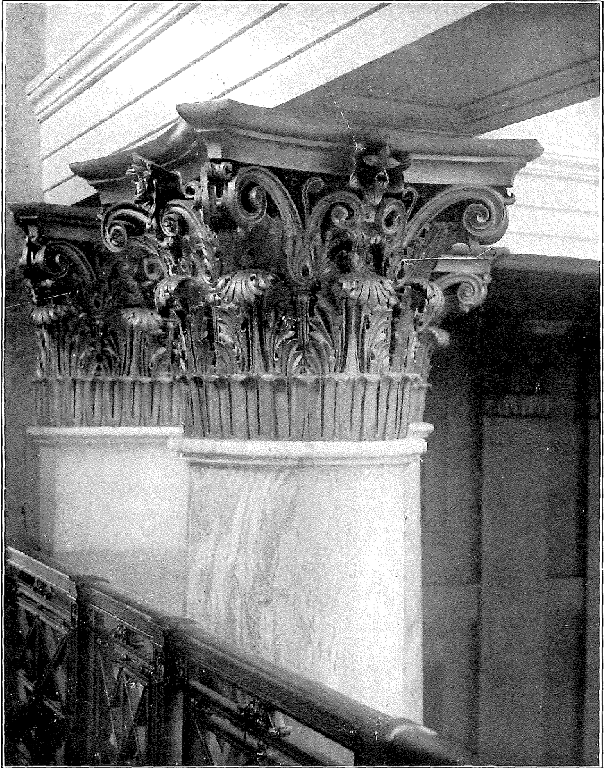
Into the beautiful Corinthian capitals which surmount the forty-four marble columns of the second floor, the architect has introduced a rosette which is a conventionalization of the moccasin plant—the recognized flower of the State of Minnesota.
