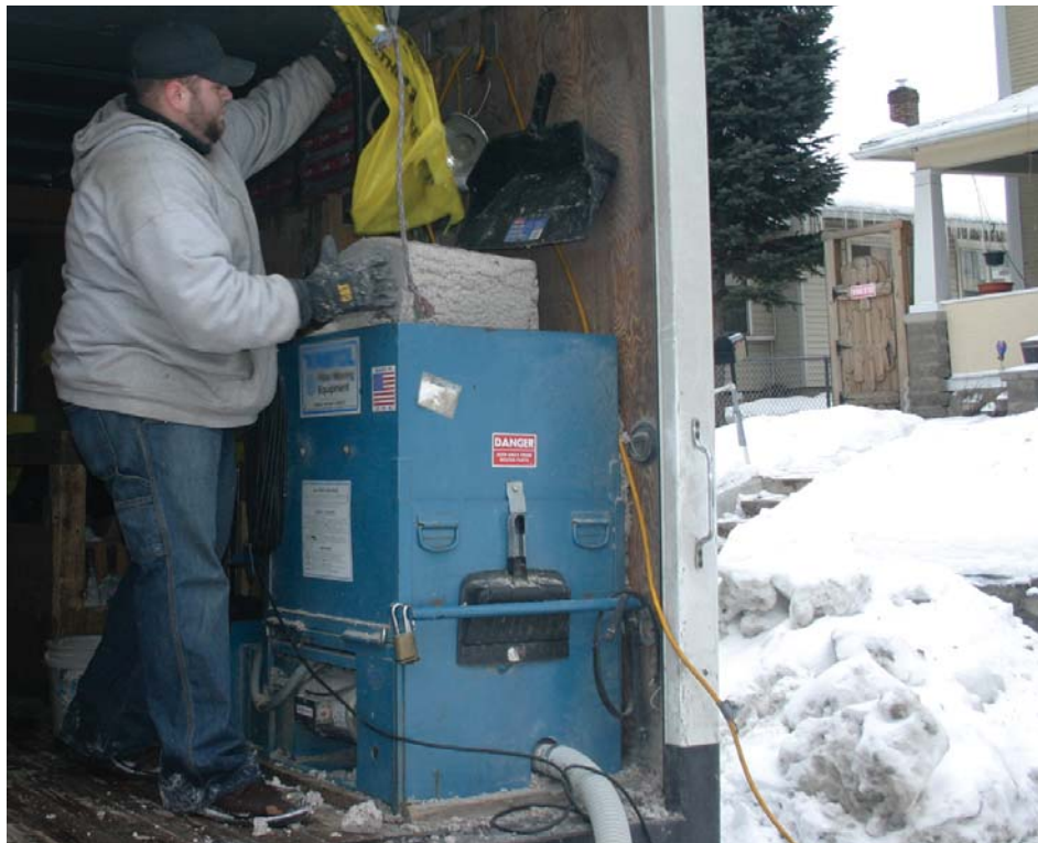
Daniel Orchard fills a blowing machine with cellulose insulation that is being dense-packed into the walls of a client's home in St. Paul.
