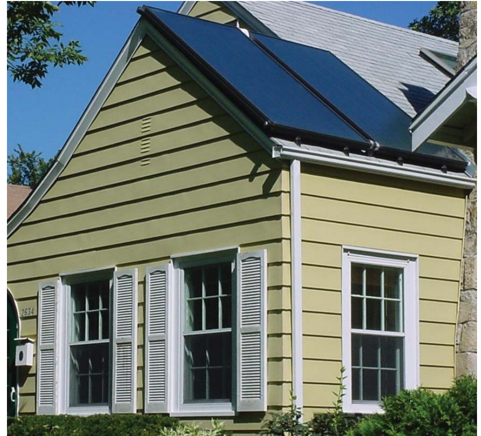
Two 4- by 8-foot solar thermal collectors are part of a closed-loop glycol thermal system that provides energy for about 75 percent of the household’s hot water needs.
