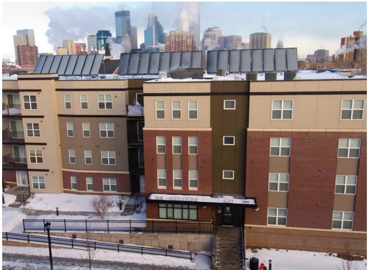
The solar thermal system for The Wellstone Apartments is exceeding expectations and meeting about 60 percent of the building's hot water needs. (Photo by Bruce Silcox Photography)
