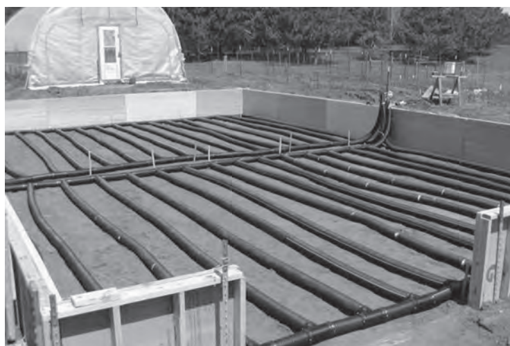
Figure 1. The lowest layer of tile line with the traditional high tunnel in the background.
