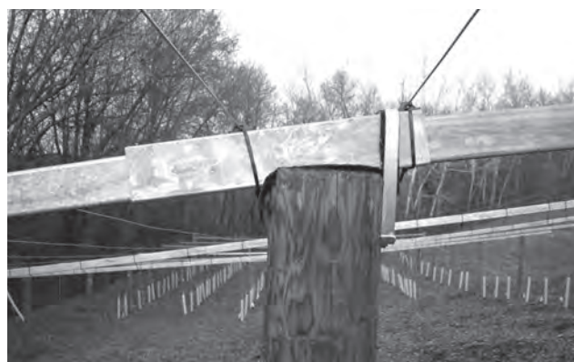
Figure 4. A joiner sleeve connects the 24' sections of galvanized tubular steel and is clamped to a notched support post. A specialized membrane prevents the steel and clamp from coming in direct contact with the wood. The overhead high-tensile wires are secured in place using nylon clips secured here to the joiner.
