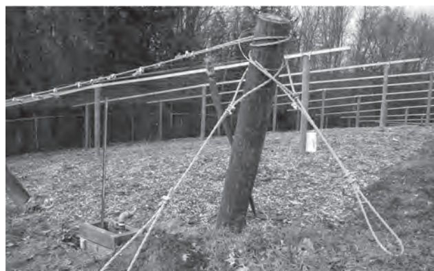
Figure 5. Two earth-anchor tiebacks stabilize each corner post and prevent it from shifting when the high-tensile wires are tensioned. Each cable is double-clamped to nearly eliminate the potential for slippage.
