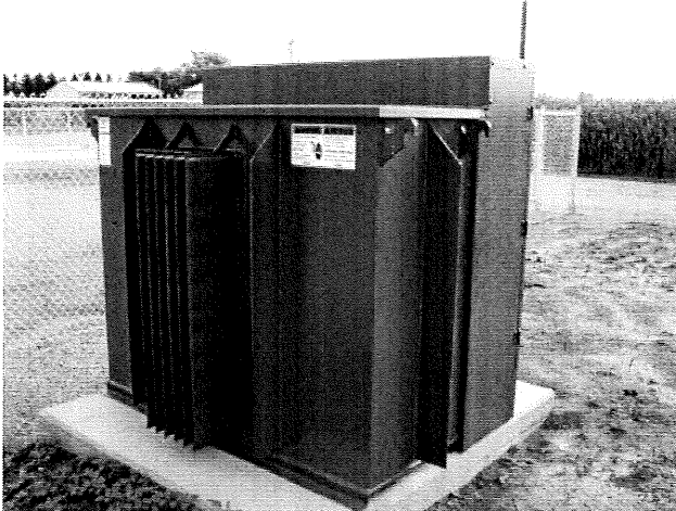
Picture 5. 12.5 kV to 480 volt transformer
