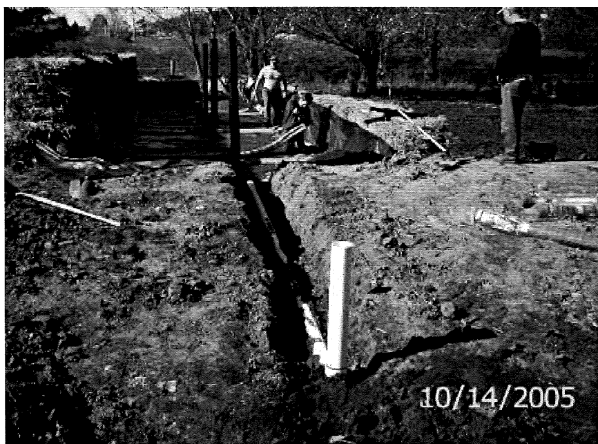
Figure 36: Front view of biofilter with intake pipe (front) and installation of "flow interceptor" H-pipes (back)
