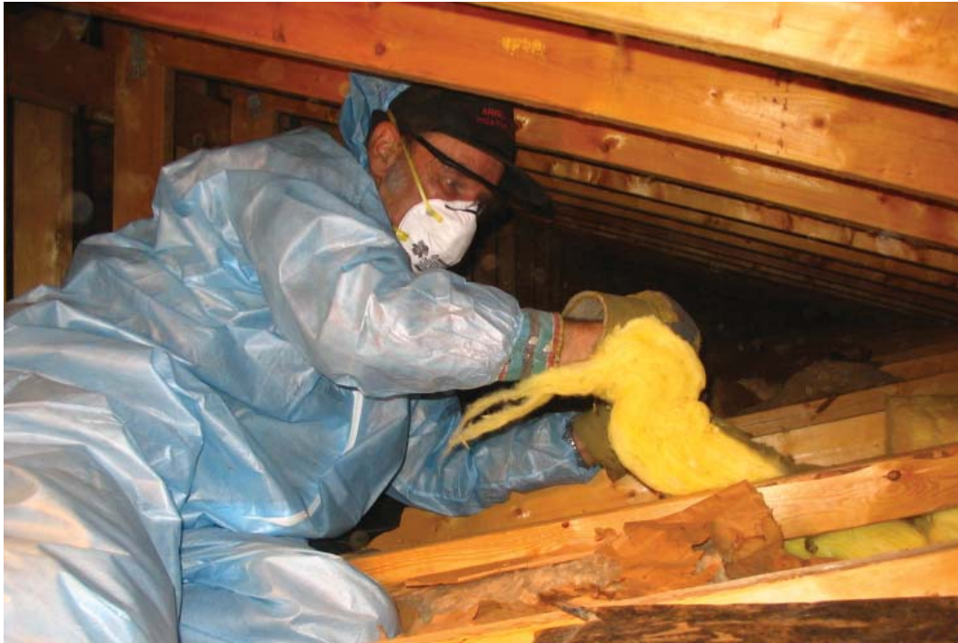
AEOA crew member Brian Leppala installs attic insulation.
