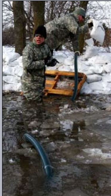
▲ Spc. Scott Nielson (left) and Spc. Dan Francis, both of A Co., 2nd Combined Arms Battalion, 136th Infantry, adjust a pump to battle a breach in a sandbag wall.
