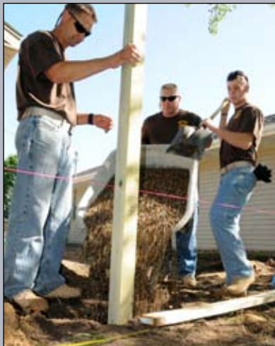
▲ Candidates Justin Smude, Todd Busswitz and Brian Nuth from the 175th Regional Training Institute position a fence post while reinforcing the hole with pea rock.
