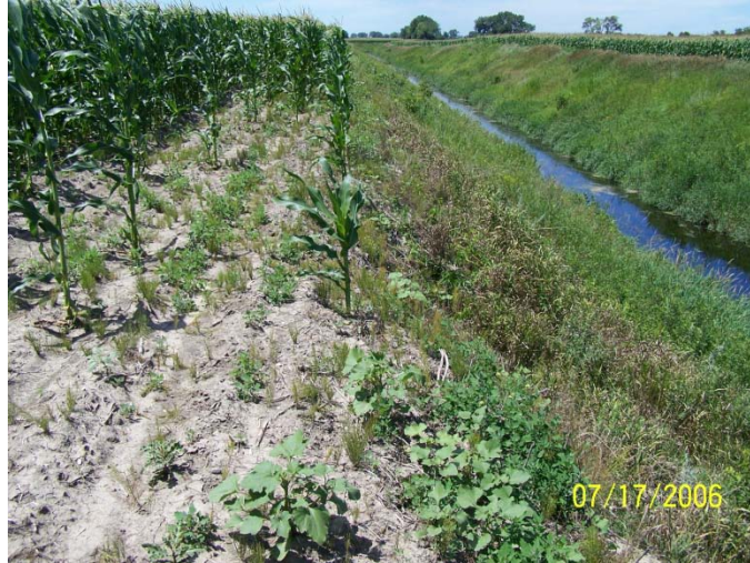
Figure 3. Drainage Ditch in Need of Buffer Strip for Tillage Setback
