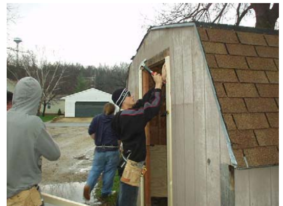
Wabasha Youthbuild, Don, applies trim to utility shed
