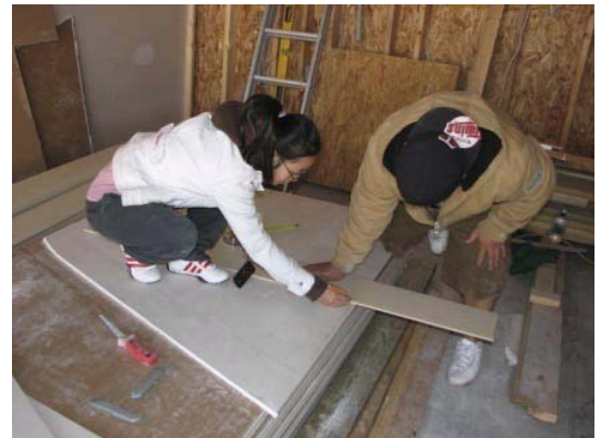
Sheet rock installation by Youthbuilders, Chantra and Fong
