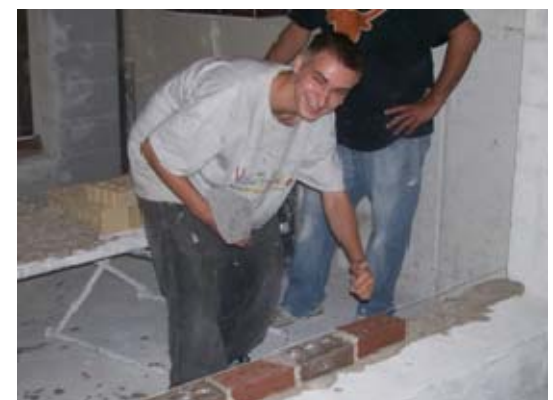
St. Cloud Youthbuilder, Blake, learns to lay bricks at the Bricklayers and Craftworkers Center in St. Paul. Each Youthbuilder is paired with an apprenticeship student for the hands-on experience.
