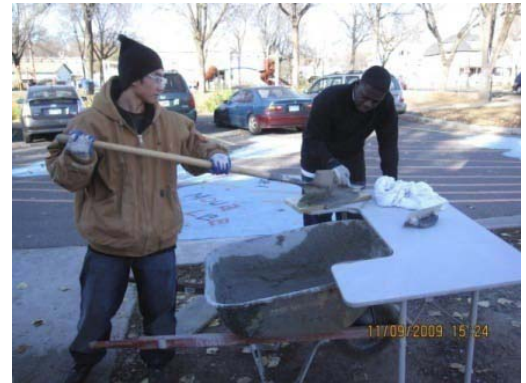
Youthbuilders Tony and Jerome mixing mortar
