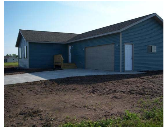
The new house built by Perham Youthbuilders to be sold as affordable housing for a low-income family
