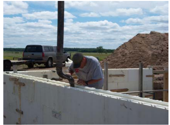
Youthbuilder inspecting plumbing during the new construction of the Perham home
