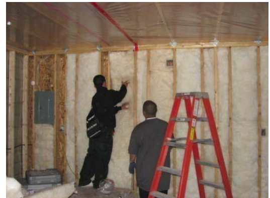
Youthbuilders, Xon and Lincoln, installing insulation
