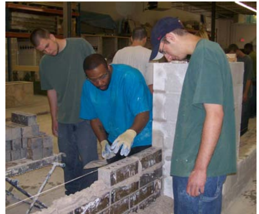
SBETC Youthbuilder laying bricks with instructor's supervision
