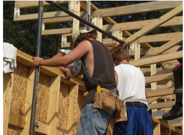
Youthbuilders framing walls on a building located in the city of Chaska
