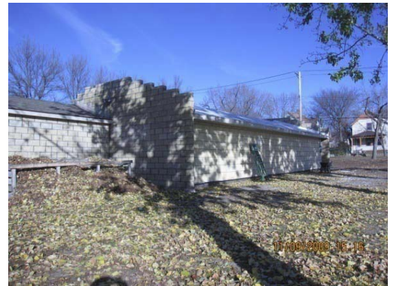
Finished garage, workshop, and compost area
