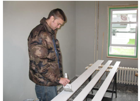
Dustin paints trim boards prior to installation during the home renovation in Chisholm
