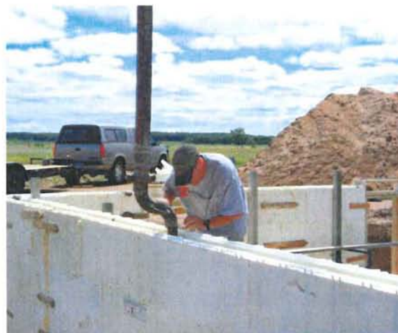
Youthbuilder inspecting the process of pouring cement between foundation forms
