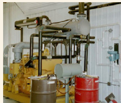
Digester engine with heat recovery system
