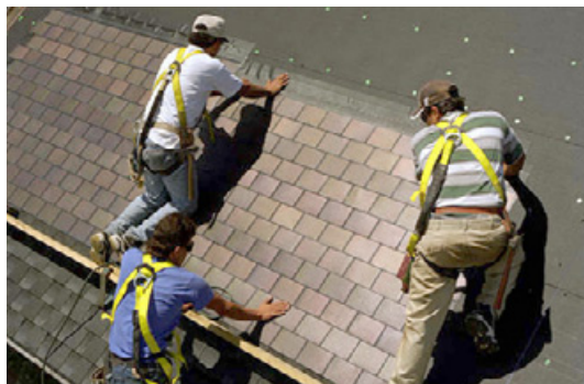
These PV shingles offer a low-profile way to add solar to a residential home
