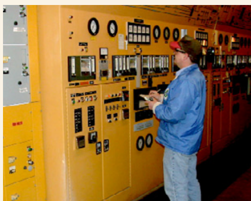
Digester controls at a wastewater treatment plant
