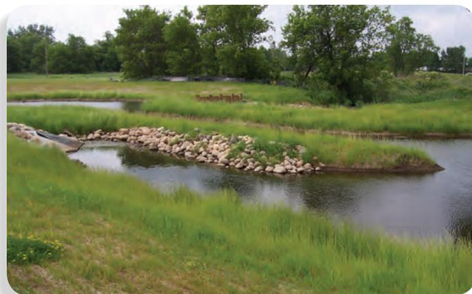
*The “S” shape of the Hickman Drive Stormwater Retention Basin provides longer retention time thus increasing sediment reduction.*
