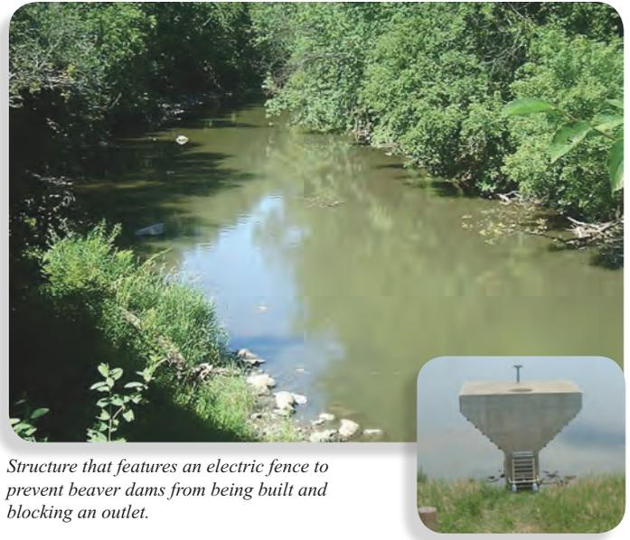
*Structure that features an electric fence to prevent beaver dams from being built and blocking an outlet.*
