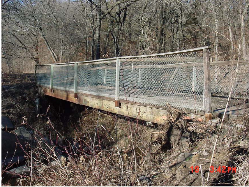
The bridge railings need to be replaced to improve safety of the Fort Ridgely Creek crossing. Photo by Bruce Eng, DNR
