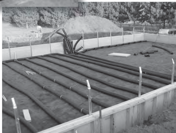
Figure 2. The second layer of tile line. The tile line was hooked up to the solar panels in the center of the picture.
