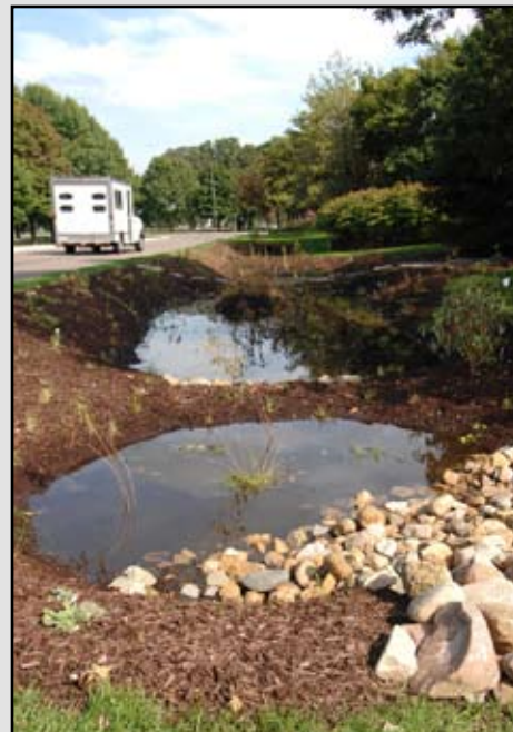
The 133rd Airlift Wing constructed the first-ever Air National Guard-funded Rain Garden. This esthetically pleasing water pollution prevention tool absorbs up to 2 ½ inches of rainfall so that runoff does not enter storm sewers.
