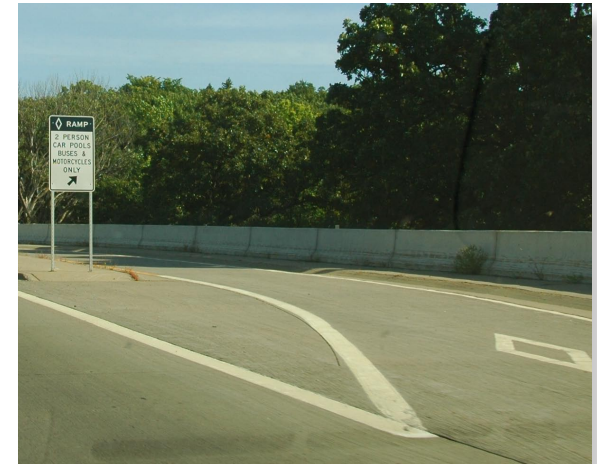
Figure 7-26: Ramp meter bypasses are transit advantages that encourage ridership by improving transit time.
